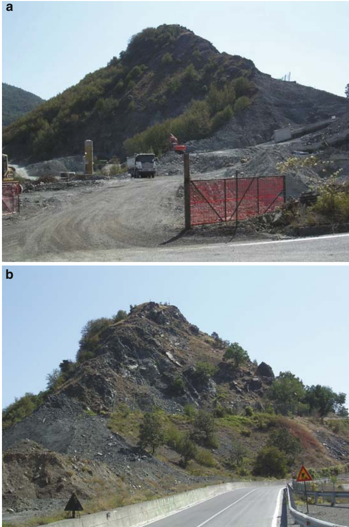
Fig. 6.9 Picture of Roccaprebalza: (a) south slope, with a widespread groundwater flow and deep instability; (b) north slope, with localized groundwater flow and superficial instability
