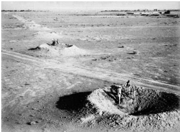
Fig. 8.4 Constructing qanats using reinforcing rings. Note the spoil crater from digging the well. (Source: Ghayour 2000)
