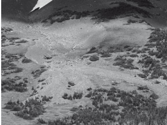
Fig. 1 The Apikuni Creek Big Red debris flow (Apikuni number 1) is evolving into a first order channel that drains the summit of Apikuni Peak. This landform has witnessed repeated debris-flow activity, with four known events since 1994. Note the impact of the channel incision on trees along the upper edges, and within the lower toe deposits
