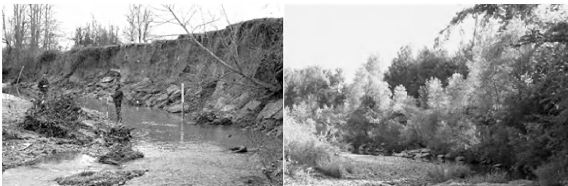
Figure 4. Views of the Goodwin Creek bendway looking downstream during (left) February 1997 (pre project) and (right) July 2009 (post project). Construction took place 26 February to 2 March 2007.
