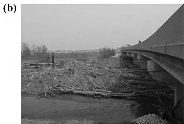
Figure 2. Debris accumulated (a) at debris deflectors upstream of bridge piers and (b) at the SR59 crossing of the Eel River, Indiana [after Lyn et al. , 2003].
