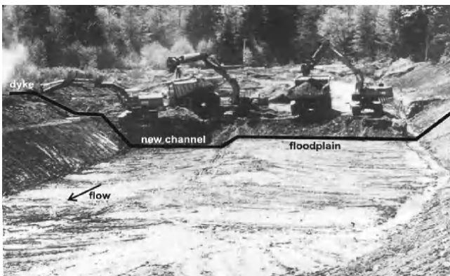
Figure 26. Channelized Oulette Creek diversion under construction in 1978.
