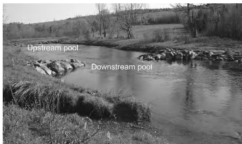
Figure 2. Upstream-oriented ( 135^\circ ) paired boulder deflectors used in the Nicolet River installed in 1997 after the unsuccessful installation of the 45^\circ wooden deflectors located farther upstream. The view is looking upstream, where the upstream paired deflectors are visible.
