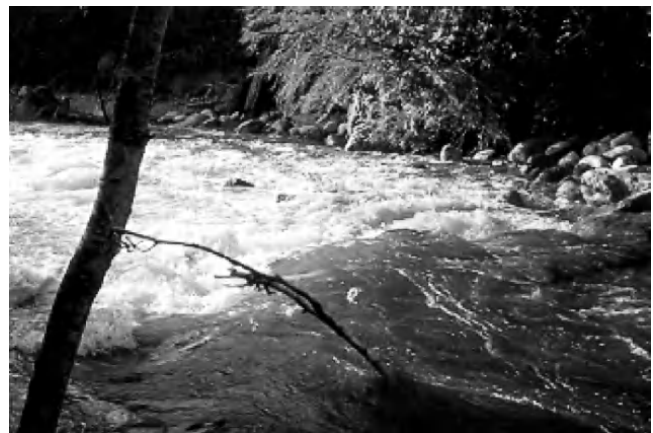
Figure 20. A rock riffle was added to Chapman Creek to retain spawning gravels and maintain water depths. The bankfull depth at the site is 1.6 m. The height of the riffle crest is 0.28 m.
