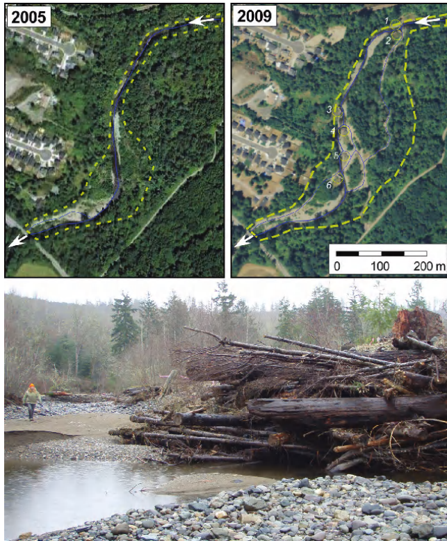
Plate 13. Project example of introducing ELJs to increase channel complexity by creating channel anabranching in the Upper Mashel River near Eatonville, Washington. Air photos of preproject (2005) and postproject (2009) conditions at restoration project constructed in 2006 and 2007 (consisting of six ELJs delineated on 2009 photo). With addition of side channels activated by ELJS, total bankfull channel length increased approximately 180% from about 890 to 1610 m. Floodplain connectivity almost doubled from about 3.6 to 6.9 ha (yellow dashed lines). The project successfully experienced a peak flow greater than 50 year recurrence flood in January 2009 with estimated velocities of over 4 \text{ m s}^{-1} and maximum shear stress of 166 Pa. Bottom photo is ELJ 2 in 2008 with side channel to left.
