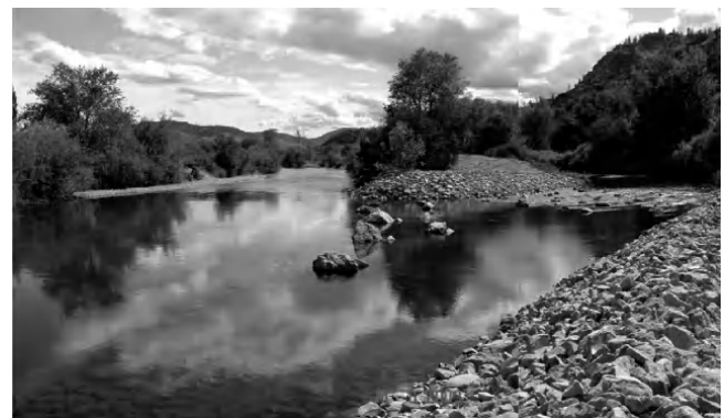
Figure 16. Entrance to upper meander bend showing spawning ramp in main stem ( Fr = 0.35 at the regulated spawning discharge of 8 \text{ m}^3 \text{ s}^{-1} ) and riffle habitat in the Loughheed meander entrance completed in August 2009.
