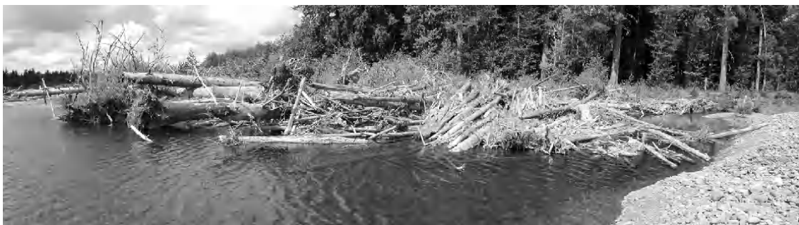
Figure 4. Wood accumulation on a constructed logjam in the Hoh River in 2008, 4 years after construction. Person in foreground gives scale of logjam. The ELJ has accumulated several thousand of pieces of debris ranging in length from 1 to over 20 m and diameters from 0.1 to 1 m. The logjam increases the surface of cover and organic substrate by over 100,000-fold.
