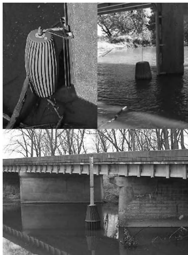
Figure 7. (clockwise from top left) Debris sweepers installed using the first-, second-, and third-generation pier attachment systems [from Sheeder and Johnson, 2008; Debris Free, Inc.].
