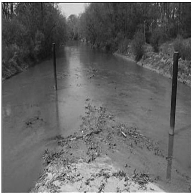
Figure 6. Debris deflectors upstream of bridge [after Bradley et al. , 2005].
