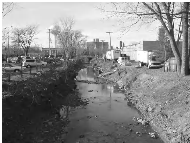
Figure 2. Parking lots and alleys flanking the WFNBCR in downtown Northbrook, November 2001.
