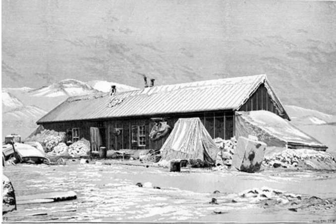
Ox House at Conger (West Side), March, 1882. (From a photograph.)
