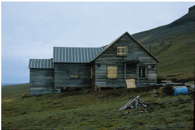
Fig. 12.5 Svenskhuset after restoration work in 1982. Photo Susan Barr
