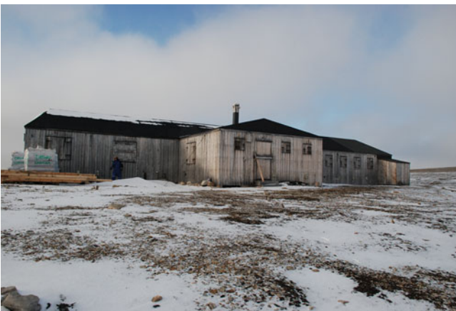
Fig. 12.11 The main Kinnvika building today. Photo Susan Barr
