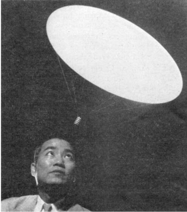
Dr Tsung-Chi Tsu of the Westinghouse Research Laboratory with a model of his proposed late-1950s solar sail spacecraft. (BIS)
