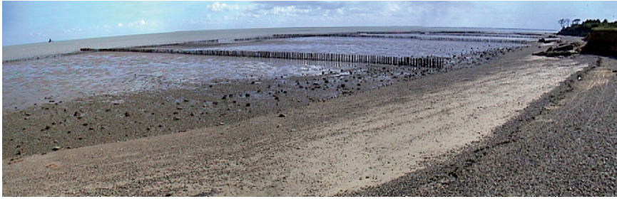
Figure 23 Wooden ‘groynes’ built on the muddy foreshore to form a polder-like structure as part of an attempt to re-create saltmarsh and prevent cliff erosion at Cudmore Grove, Mersea Island, Essex. Monitoring showed that by 1990 (some 14 months after installation) Spartina anglica , present when construction took place, was still there. There was also some evidence of accretion in sheltered parts of the polder. However, by 2002 as the above picture shows, there were no signs of saltmarsh development
