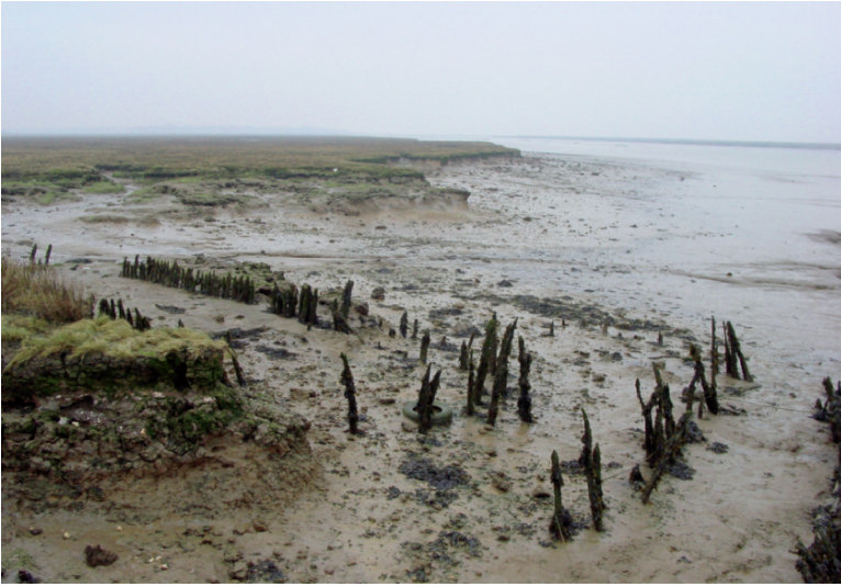
Figure 22 Loss of saltmarsh on the Essex coast, south-east England. Note, as erosion proceeds, exposure of previous attempts to stabilise the saltmarsh occurs
