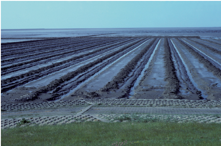
Figure 45 Parallel lines of excavated ditches enclosed by brushwood fences, designed to encourage saltmarsh development seaward of a sea wall in the Danish Wadden Sea, 1992. Note excavated ridges to encourage vegetation
