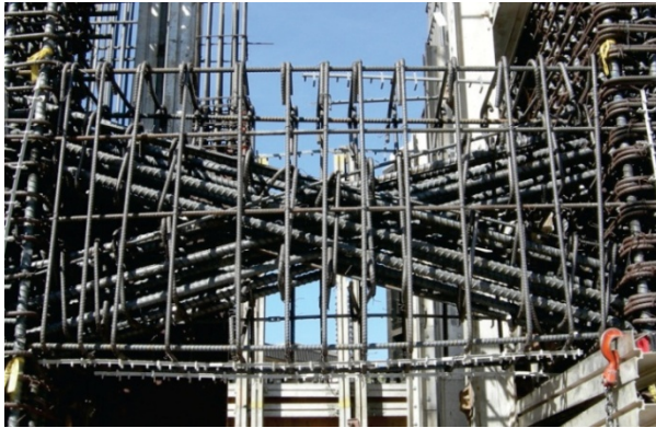
Fig. 1. Reinforcement detailing in diagonally reinforced coupling beam
