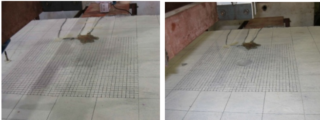
Fig. 5. Damage development of ECC 100 panel on impact face at 1 st impact (left) and at 10 th impact (right)
