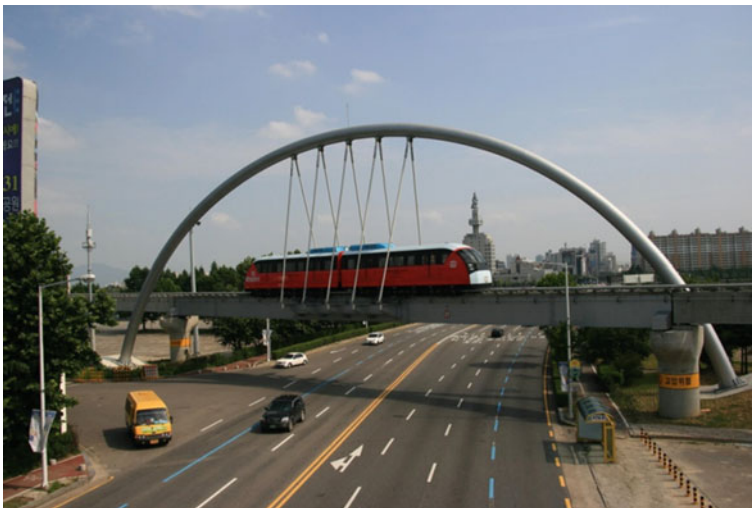
Fig. 5.80 EMS type vehicle running over a long span elevated guideway
