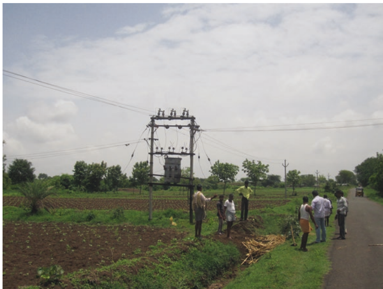
Fig. 2.4 Farmers collectively repairing their DTR. Source Christian Kimmich
