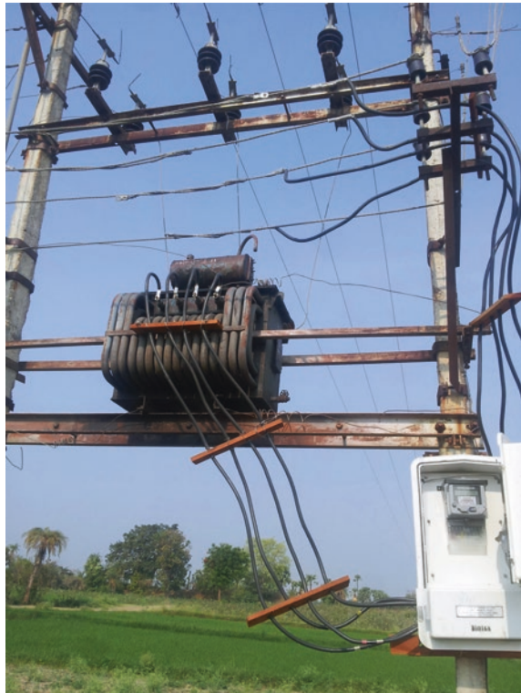
Fig. 4.1 Agricultural DTR with meter in Andhra Pradesh, Source Malte Müller
