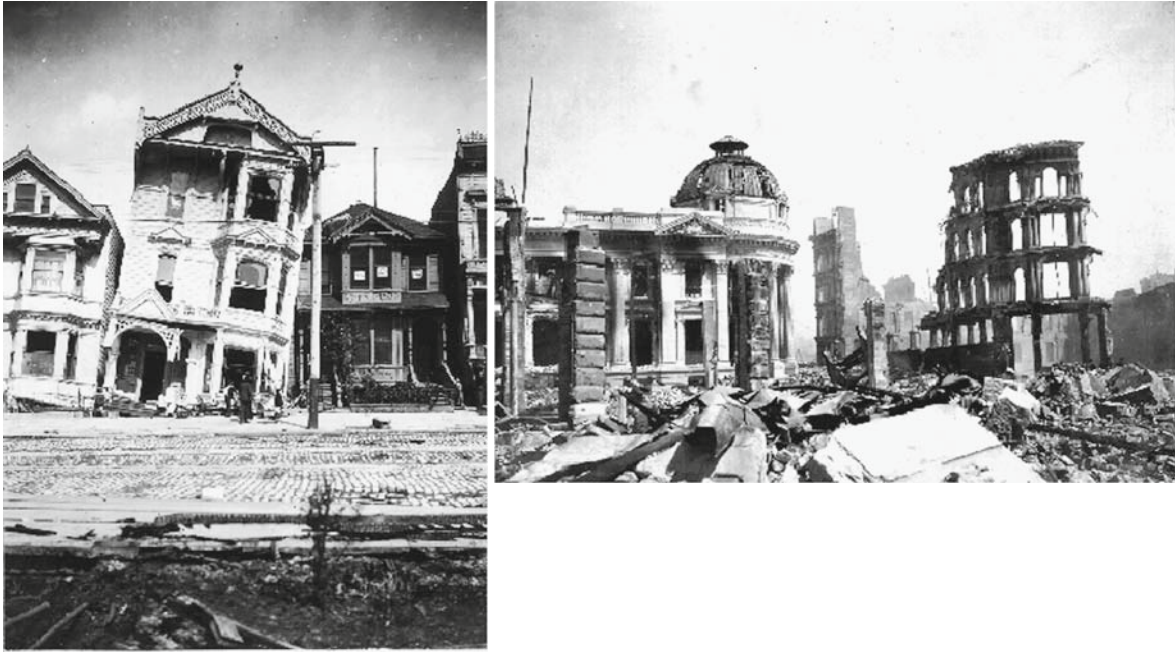
Fig. 7 Photographs taken after the 1906 Great San Francisco earthquake and fire. Left: damage to houses on the east side of Howard Street near Seventeenth Street. Right: The remains of the
