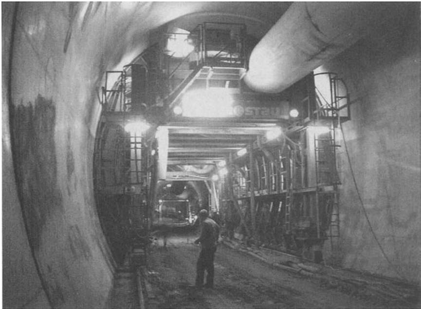
Figure 4.9 Formwork for cast concrete secondary lining
