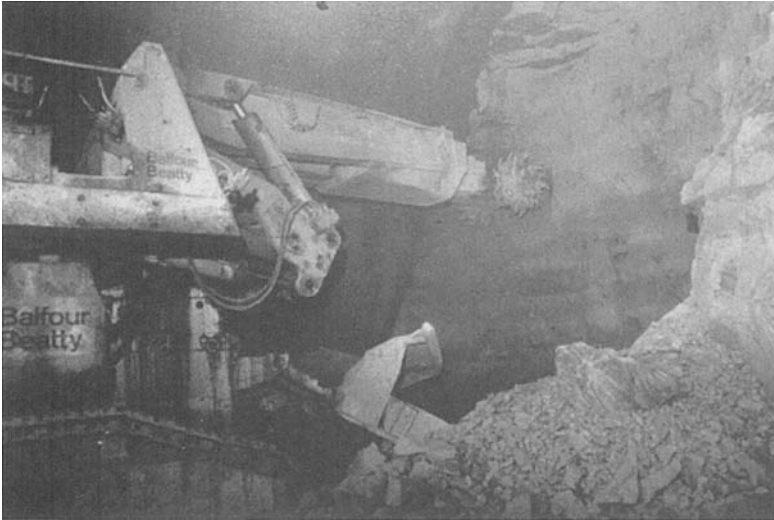
Figure 3.6 Excavation of a SCL tunnel using a roadheader
