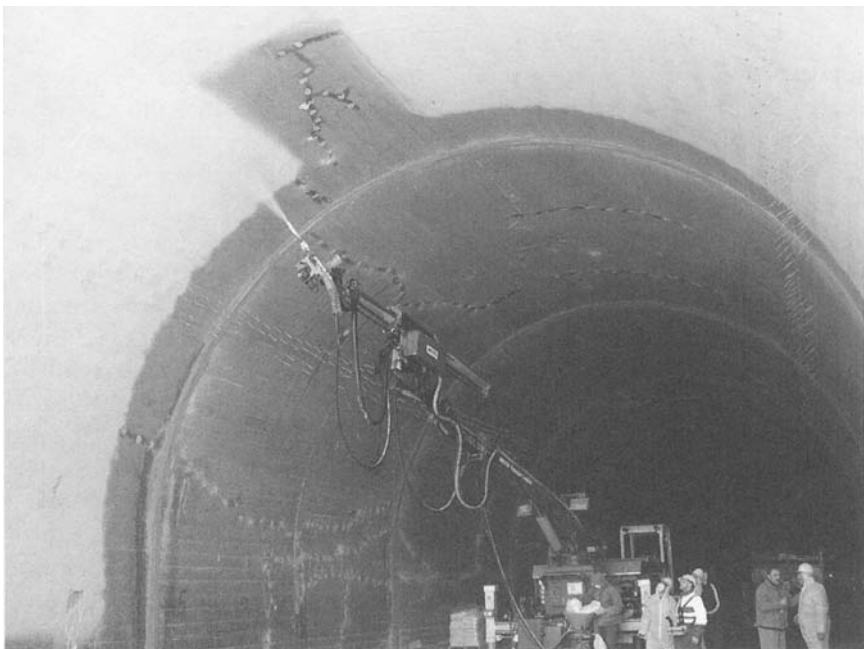
Figure 4.8 Spray-on membrane installation (courtesy of BASF)
