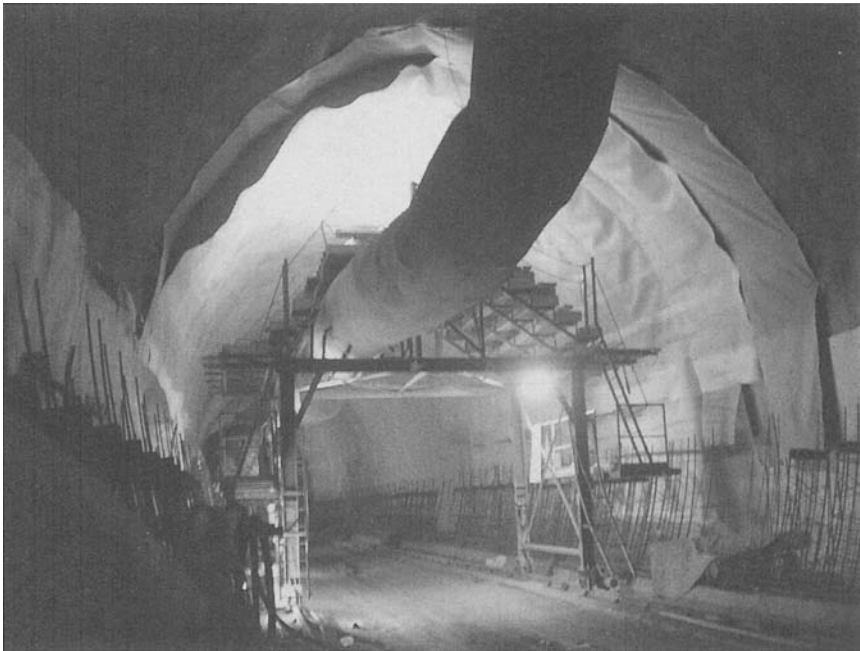
Figure 4.6 Sheet membrane installation
