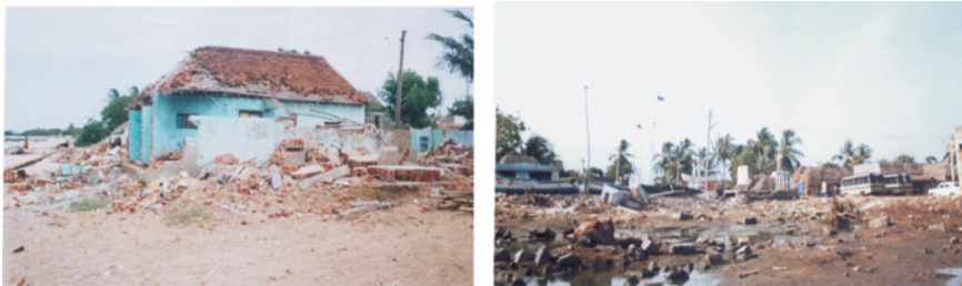
Figure 2: Destruction of houses built on sand dunes in coastal villages.
