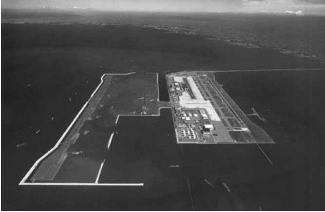
FIGURE 1.4 Kansai International Airport during phase II construction in 2002. (Photo courtesy of Kansai International Airport Land Development Co.)
