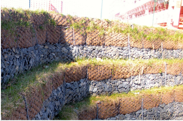
Figure 16.10 “Green” gabion wall. Courtesy of Maccaferri, Inc.
