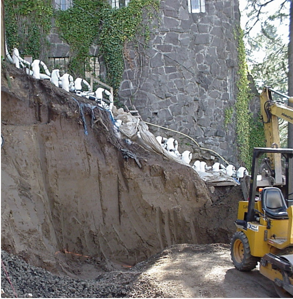
Figure 13.9 Freezing for excavation adjacent to sensitive historic structure. Courtesy of SoilFreeze.
