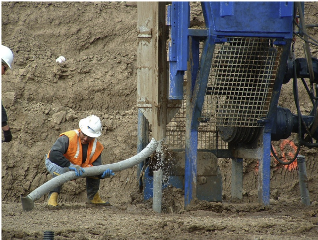
Figure 8.9 Earthquake drain installation. Courtesy of HB Wick Drains.
