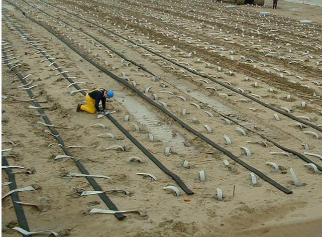
Figure 9.7 Horizontal strip drain discharge system connected to PVDs. Courtesy of Hayward Baker/HB Wick Drains.
