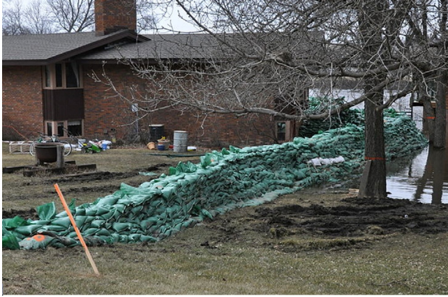
Figure 16.1 Use of sandbags as a temporary “earthen” flood control levee. Courtesy of FEMA.
