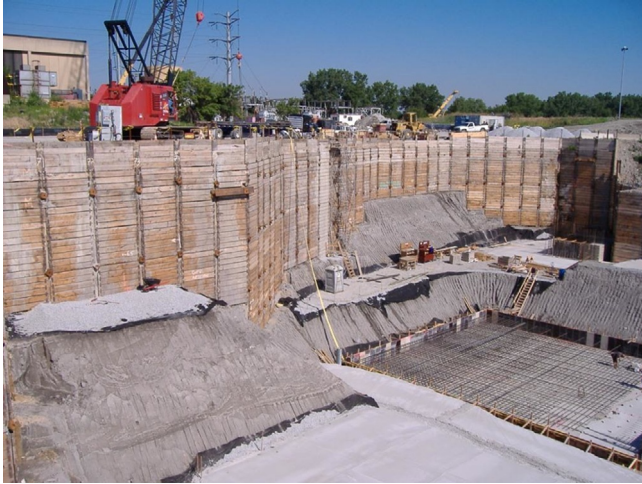
Figure 16.4 Photo of a soldier piles and lagging excavation support. Courtesy of Hayward Baker.
