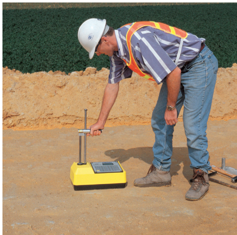
Figure 5.22 Field operation of a nuclear gauge. Courtesy of Troxler Laboratories.
