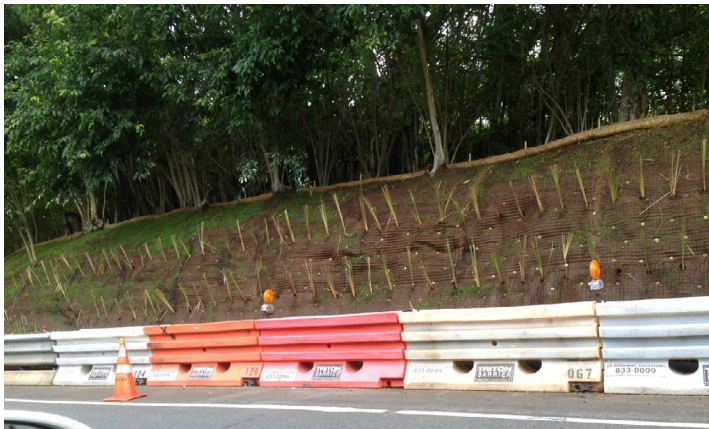
Figure 14.30 Reinforced steep slope surface with vegetation “plugs.”
