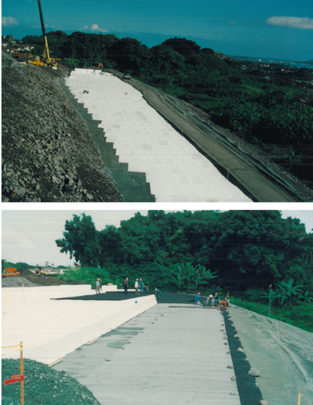
Figure 17.19 Highway embankment construction, Kaneohe, Hawaii. Courtesy of Geolabs Hawaii.
