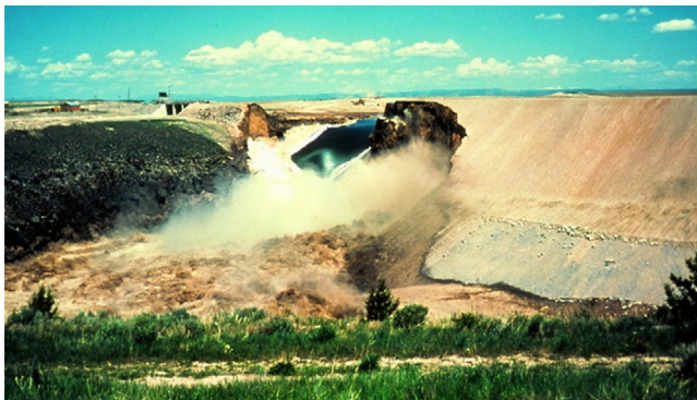
Figure 3.12 Failure of the Teton Dam, June 1976. Photo by Mrs. Eunice Olsen.
