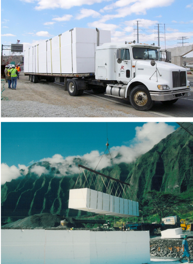
Figure 17.7 Bulk Geofoam site delivery. Top courtesy of FHWA; bottom Courtesy of Geolabs Hawaii.
