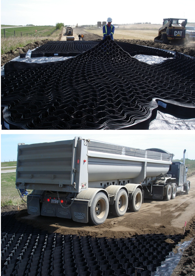
Figure 16.14 Cellular confinement for rapid construction of high capacity unpaved roads. Courtesy of Presto Geosystems.
