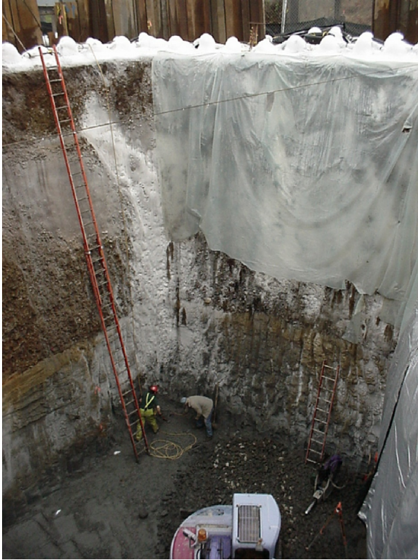
Figure 13.2 Frozen ground for excavation shoring. Courtesy of SoilFreeze.
