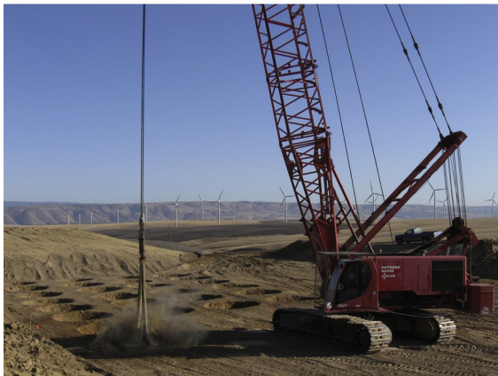
Figure 6.13 Photos of DDC field applications. Courtesy of Hayward Baker (top) and Densification, Inc. (bottom).
