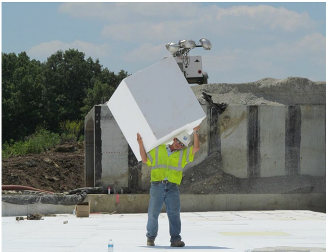
Figure 17.6 Minimal labor force needed for Geofoam installation. Courtesy Atlas EPS.
