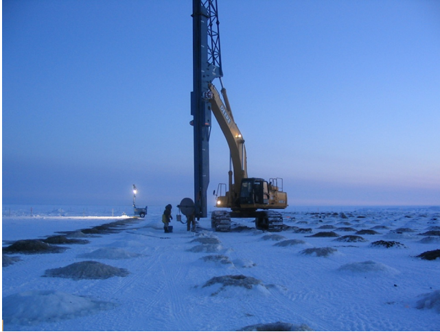
Figure 9.9 PVD install through Arctic ice. Courtesy of Hayward Baker/HB Wick Drains.
