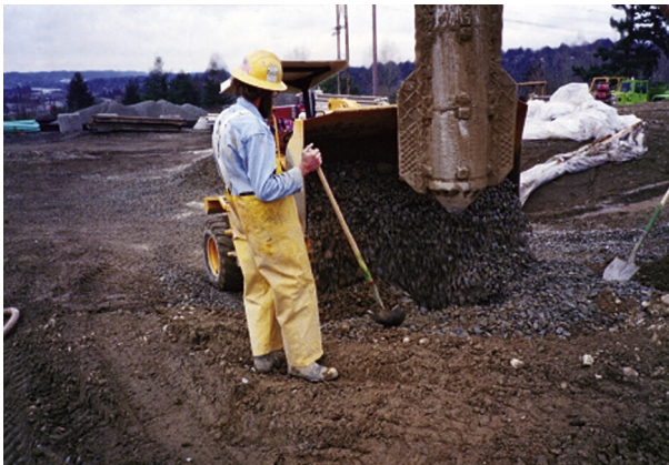
Figure 6.6 Stone column field application. Courtesy of Hayward Baker.
