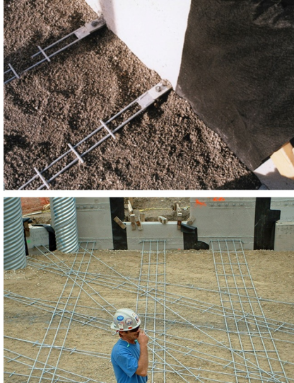
Figure 14.3 Welded wire bars and mats used for MSE wall reinforcement. Courtesy of The Reinforced Earth Company.
