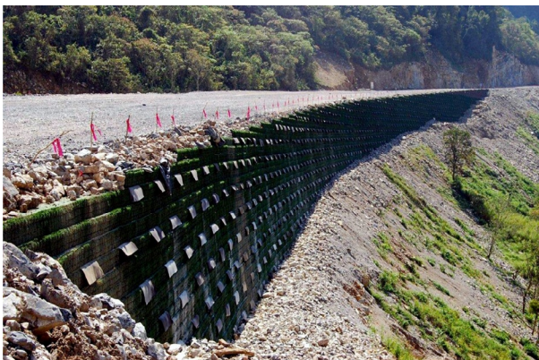
Figure 14.12 Geosynthetic wrapped-face wall. Courtesy of Tencate-Mirafi.
