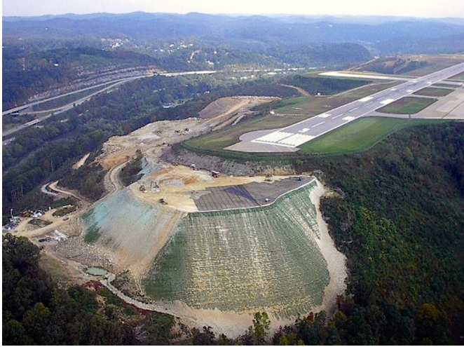
Figure 14.19 Steep, high reinforced soil slope for runway extension. Courtesy of Tecate-Mirafi.
