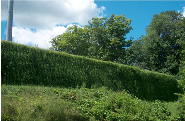
Figure 16.20 Composite geocell wall before and after vegetation. Courtesy of Presto Geosystems.
