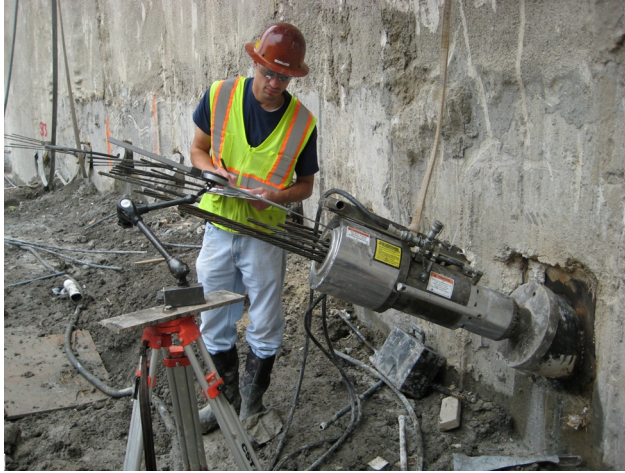
Figure 15.12 Multistrand ground anchor testing. Courtesy of Hayward Baker.
