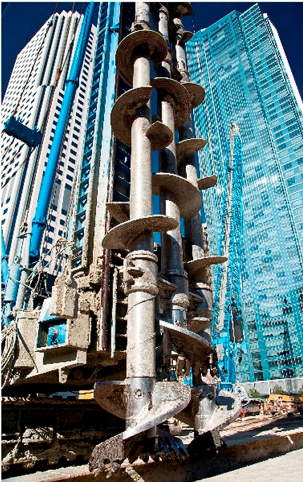
Figure 11.11 Multi-axis deep soil mixing equipment. Courtesy of Malcolm Drilling.
