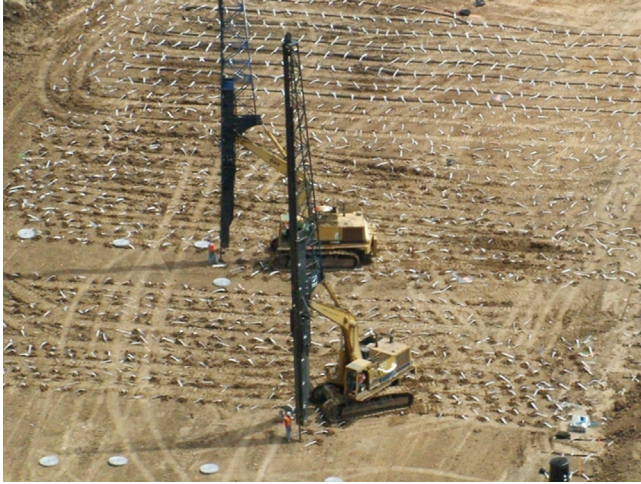
Figure 9.6 Photo of PVD installation. Courtesy of Hayward Baker/HB Wick Drains.
