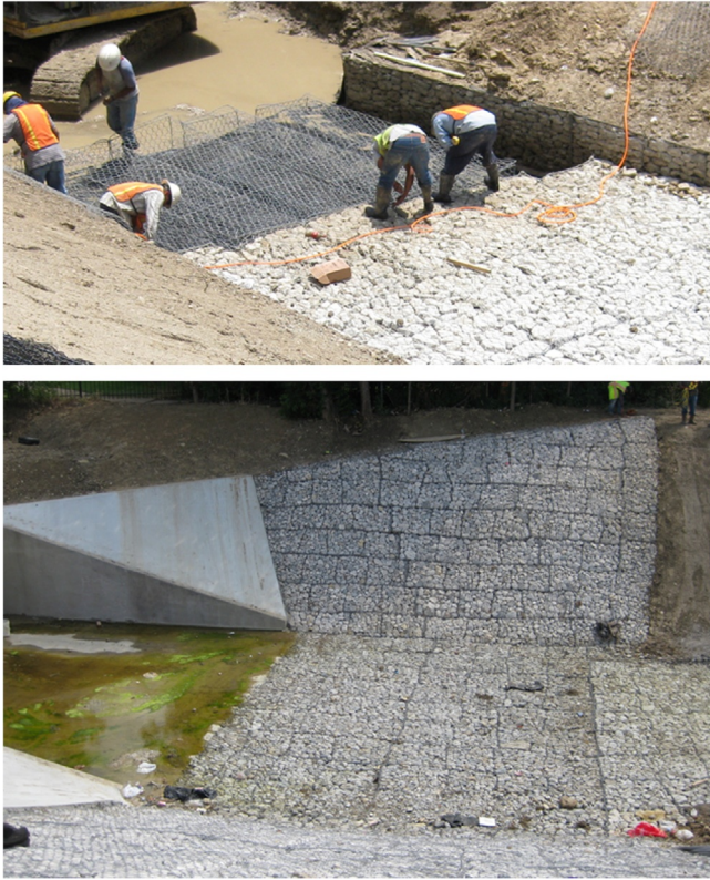
Figure 16.11 Gabion mattress for channel lining. Top: Courtesy of Maccaferri, Inc.; Bottom: Courtesy of Tensar International Corporation.
