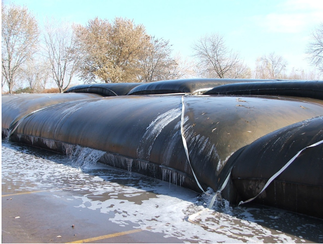
Figure 8.2 Dewatering of dredged sediment with Geotubes. Courtesy of Infrastructure Alternatives.
