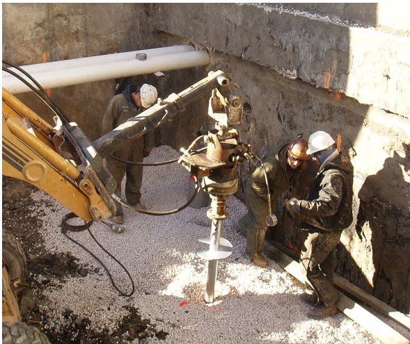
Figure 15.15 Installation of a helical pier. Courtesy of Hayward Baker.
