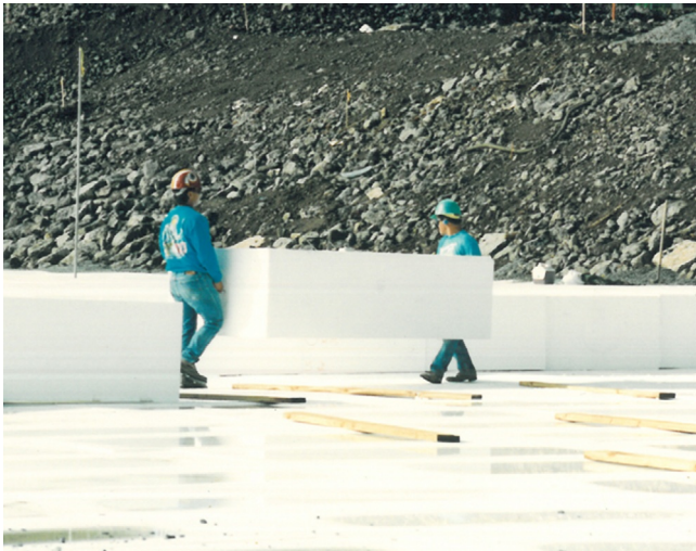
Figure 17.1 Geofoam blocks. Courtesy of Geolabs Hawaii.
