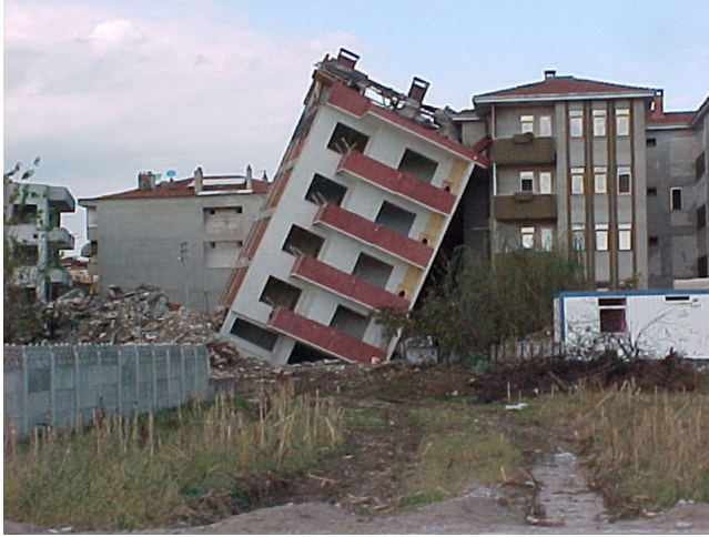
Figure 3.9 Liquefaction-induced bearing capacity failure. Courtesy of GEER.
