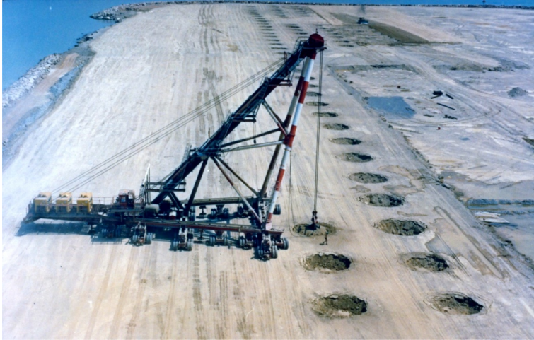
Figure 6.15 Menard's "Giga" compactor drops a 200 ton weight. Courtesy of Menard.
