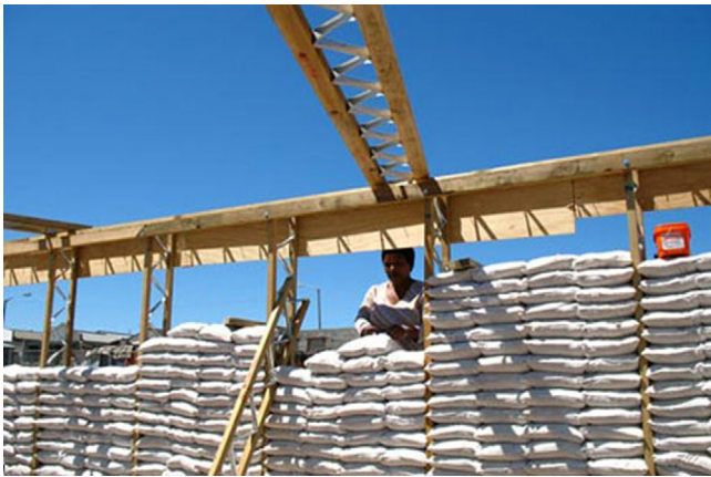
Figure 16.2 Low-cost, sandbag home construction in South Africa ( www.architecturalist.com ).
