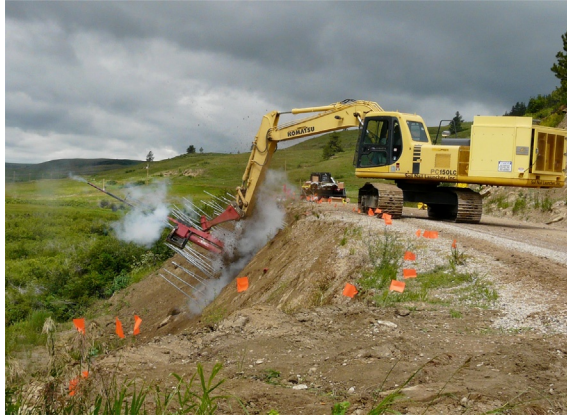
Figure 15.6 Launched soil nails for emergency slope stabilization. Courtesy of GeoStabilization International.
