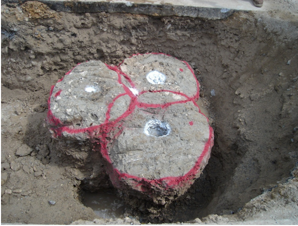
Figure 12.8 Overlapped jet grout columns. Courtesy of Yogi Kwong Engineers.
