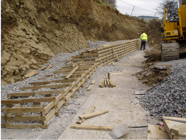
Figure 16.6 Crib wall under construction. Courtesy of Maccaferri, Inc.
