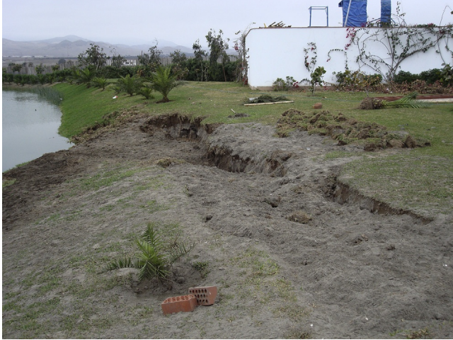
Figure 3.11 Liquefaction-induced lateral spreading. Courtesy of GEER.
