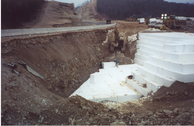
Figure 17.4 Example of Geofoam for fill of transportation projects. Courtesy of AFM Corporation.
