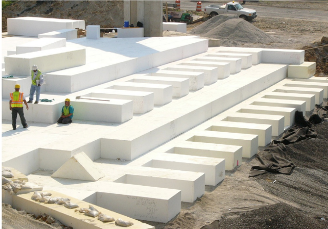
Figure 17.10 Staggering of blocks for stability. Top courtesy of AFM Corporation; bottom Courtesy of FHWA.
