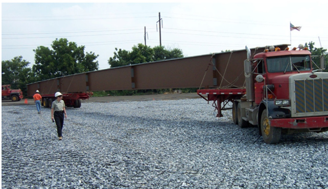
Figure 16.16 Very high load capacity gravel-filled geocells. Courtesy of Presto Geosystems.
