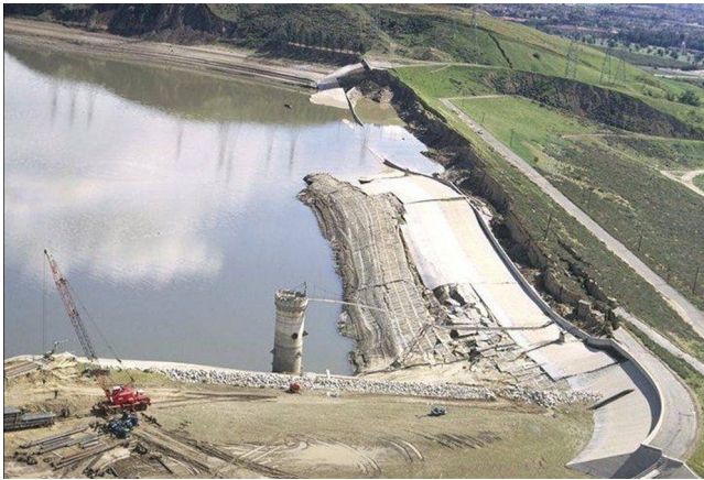
Figure 3.10 Liquefaction-induced slope stability failure, San Fernando Dam. Courtesy of EERC.
