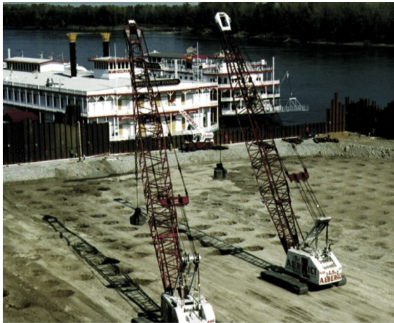
Figure 6.12 Schematic of deep dynamic compaction (DDC). Courtesy of Densification, Inc.
