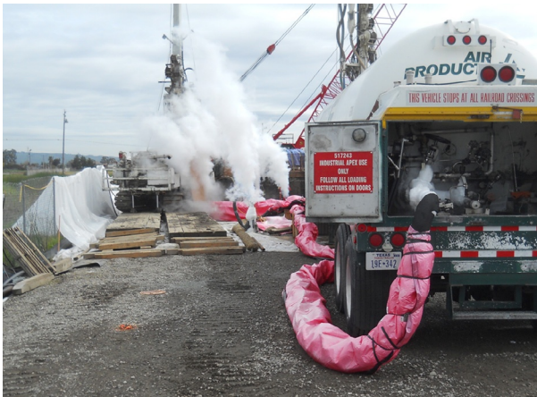
Figure 13.7 Application of freezing by injecting liquid nitrogen. Courtesy of SoilFreeze.
