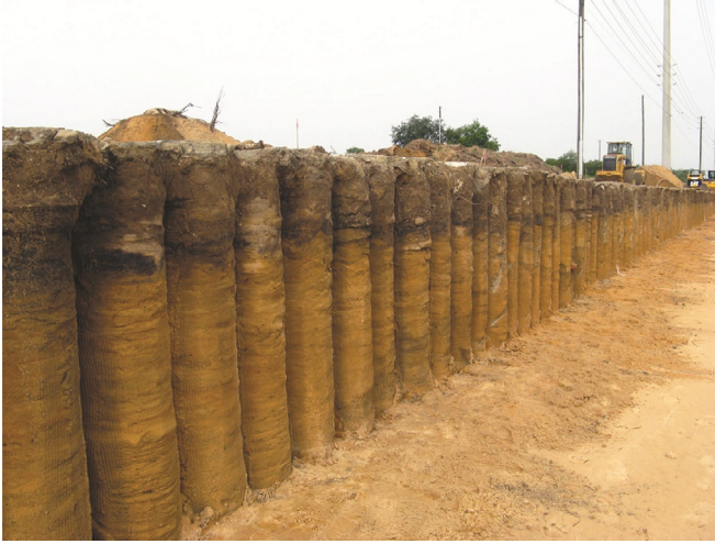
Figure 11.13 Excavated soil-lime column wall. Courtesy of Hayward-Baker.
