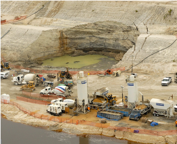
Figure 12.17 Compaction grouting to remediate large sinkholes. Courtesy of Moretrench.
