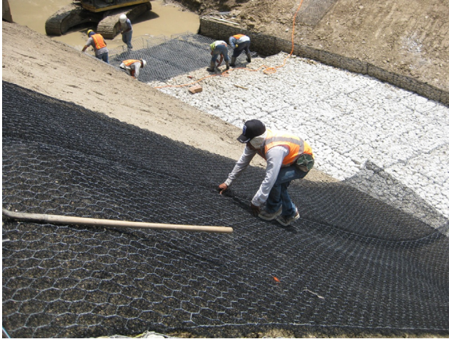
Figure 16.28 High-strength erosion control mat installation. Courtesy of Maccaferri, Inc.
