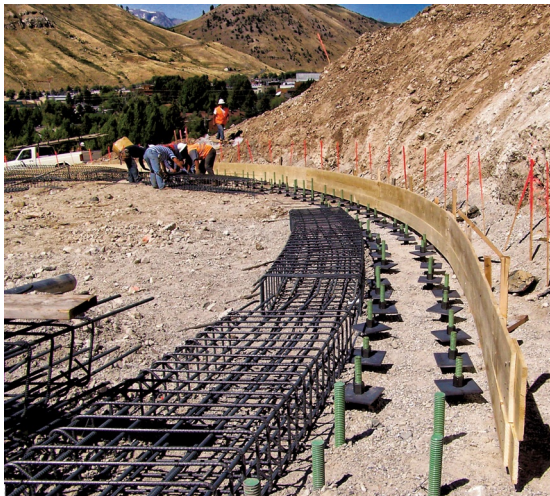
Figure 15.10 Minipiles (vertical soil anchors) for roadway support. Courtesy of GeoStabilization International.
