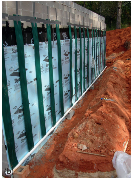
Figure 8.12 Typical installations of micro-siphon drains. (a) Horizontal installation. (b) Vertical wall installation. Courtesy of Smartdrain.
