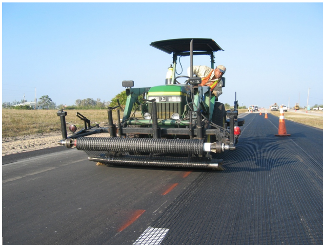
Figure 14.24 Biaxial geogrid for pavement support. Courtesy of Tensar International Corp.
