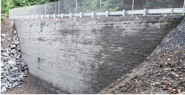
Figure 16.26 Geosynthetically confined soil (GSC/GRS) supporting a roadway. Courtesy of GeoStabilization International.
