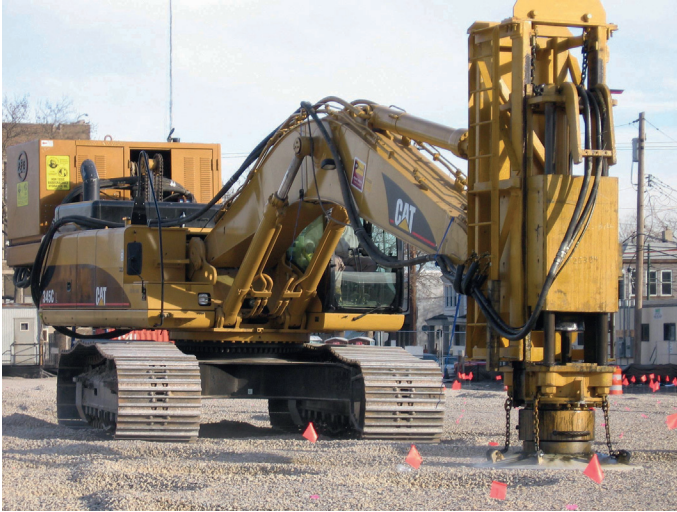
Figure 6.16 Rapid impact compaction field application. Courtesy of Hayward Baker.
