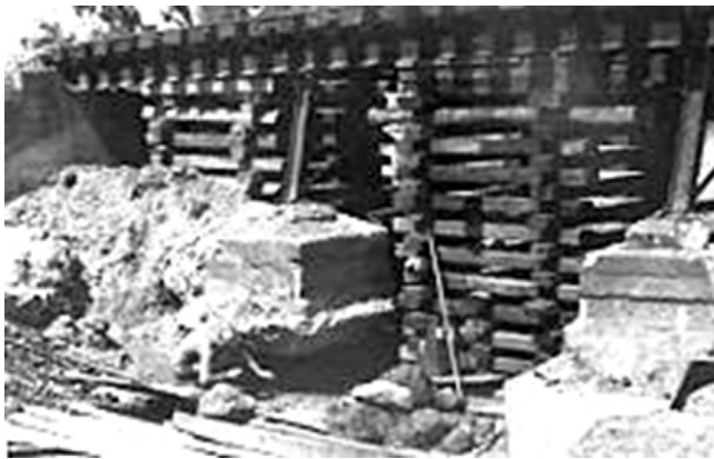
Figure 16.5 Historic use of cribs for railroads. Image by Bill Bradley.
