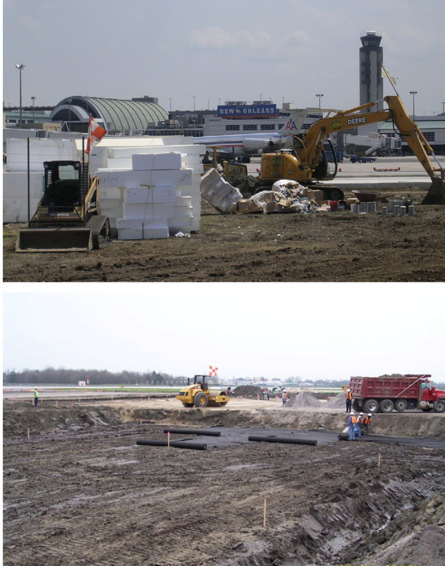
Figure 17.18 Geofill application for expanded taxiway at Louis Armstrong International Airport, New Orleans, LA. Courtesy of AFM Corporation.
