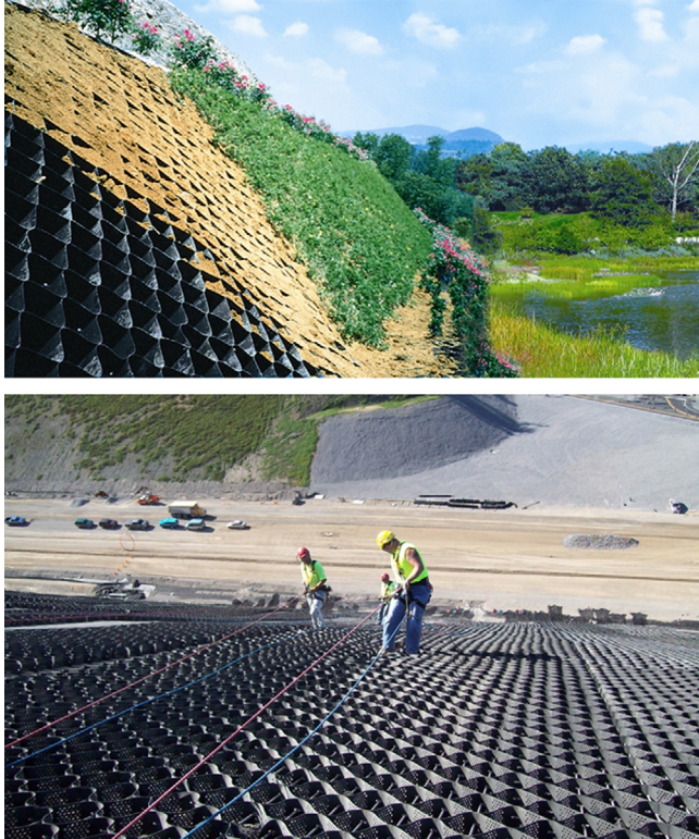
Figure 16.23 Cellular confinement (geocells) for stabilization of surface soils on steep slopes. Courtesy of Presto Geosystems.
