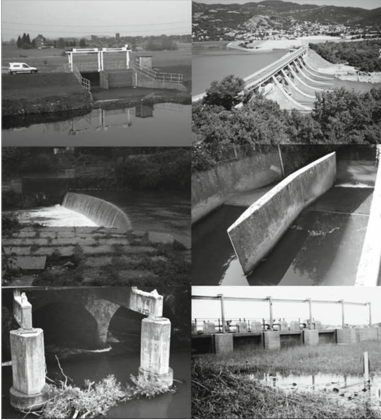
Fig. 9.1 Illustration of some types of river structures, clockwise from top left (a) sluice gates at off-line storage area (England) (b) hydropower scheme (France) (c) compound Crump Weir gauging structure (England) (d) irrigation canal sluice gates (Somalia) (e) arched culverts (England) (f) weir (Wales). Credits: (a) Sene (2008); (c) Copyright © Environment Agency 2009, all rights reserved
