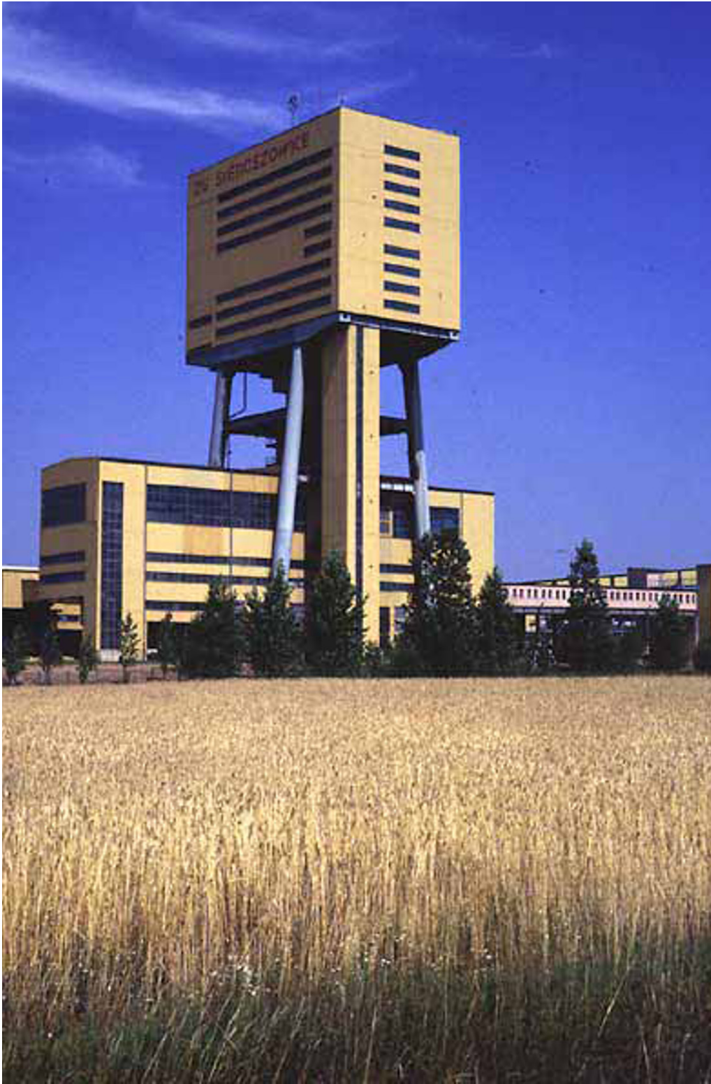
Polish Kupferschiefer district, Sierszowice Mine shaft near Lubin hauling copper ore from 1,000 m depth (PL 1994)
