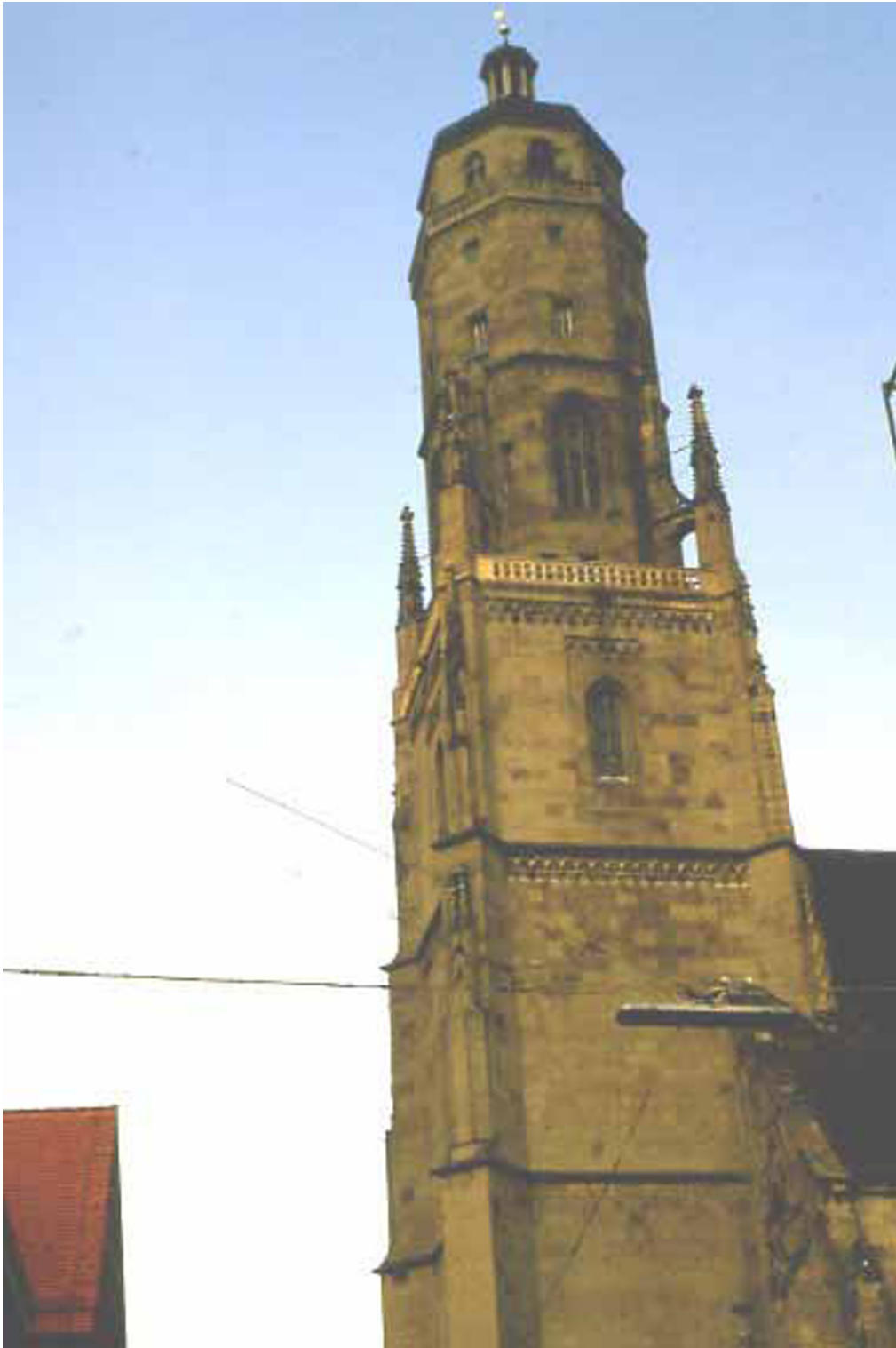
Sankt Georgkirche, Nördlingen, Bavaria, in the Ries Tertiary impact crater, constructed entirely from meteorite fallback breccias
