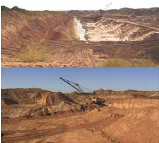
Figure 13.10. Nikopol, dragline mining of the Mn bed from depths of 20–30 m under unconsolidated overburden. PL 8-2006
