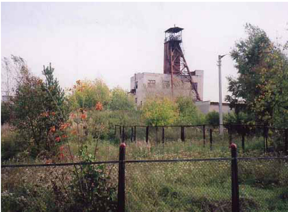
Two historic vein deposits: Montevecchio-Pb, Zn, Ag in SW Sardinia, Italy (top) and one shaft in the Berezovskii goldfield near Yekaterinburg, Urals, Russia. Both were high-labor, low-volume underground operations prevalent before the onset of large-volume, bulk mining from open pits. Montevecchio is depleted and developed into a historical park, Berezovskii goldfield still has several operating mines. PL 2006, 2008.
