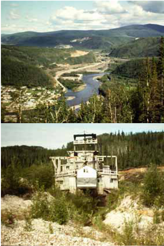
Figure 13.56. Klondike valley near its entry into Yukon River (Dawson City is at bottom left) showing gravel dumps remaining after dredging of valley gold placers in the 1930s (after thawing the permafrost!) as well as the lower Au grade Tertiary terrace gravels preserved at hillslopes above the valley (top center). Bottom picture shows one of the grounded and abandoned dredges. PL 1975
