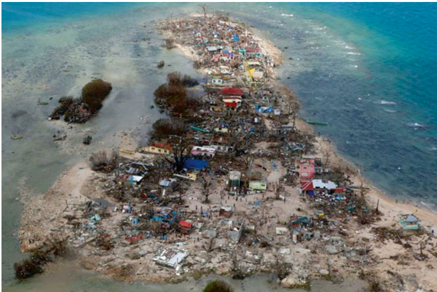
Fig. 1.15 It is not just the wind that causes the devastation but the storm surges and flooding associated with these super storms. Super Typhoon Haiyan was particularly devastating due to the low lying land and islands that makes up much of the Philippines. Source: Reuters. Reproduced under licence Reuters Thompson
