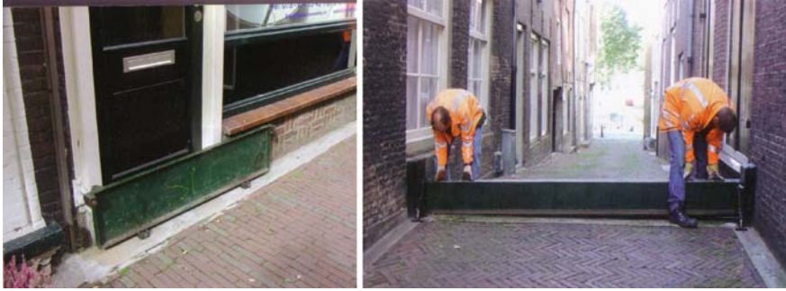
Fig. 4.23 Dry proof house measures outside the house keep the house dry (Source: www.waterbestendigbouwen.nl )
