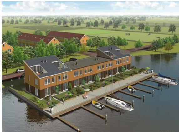
Fig. 4.26 Floating houses (Source: Dura Vermeer Business Development)
