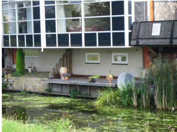
Fig. 4.24 Shore house, Amersfoort (Source: www.waterbestendigbouwen.nl )
