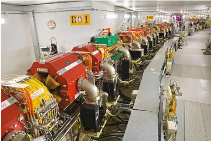
Fig. 5.16 The lattice of the UK Diamond Light Source storage ring, showing the pattern of dipole (in green), quadrupole (in red) and sextupole (in yellow) magnets (coloured online). © Diamond Light Source printed with permission
