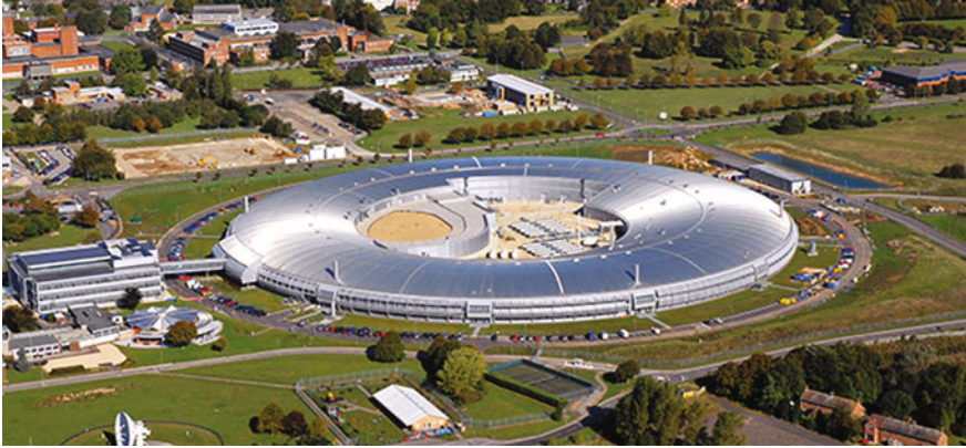
Fig. 5.11 Aerial view of the UK Diamond Light Source. © Diamond Light Source, printed with permission from [11]
