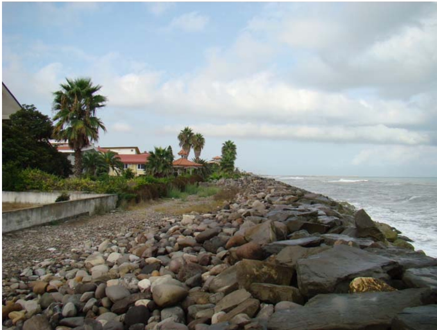
Fig. 8 Sea wall along the Mazandaran coast, at Babolsar, Mazandaran University's residential campus. The sea wall protected the campus against sea level rise and coastal retreat. Photograph by Majid Shah-Hosseini (2007)
