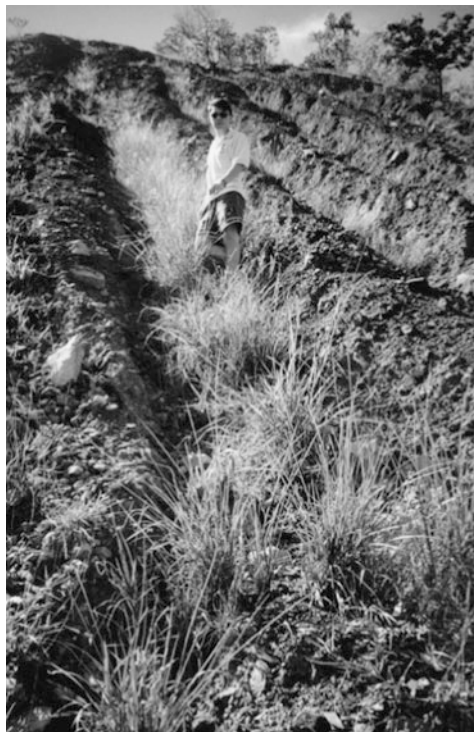
Fig. 8.11. Vetiver applications on coal mine overburden. Vetiver was planted in the gullies to stop further erosion and to encourage the re-establishment of native species. Excellent growth was obtained 6 months later.
