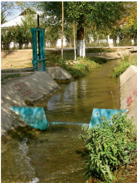
Fig. 5.4 Irrigation canal in the Jalal-Abad oblast of southern Kyrgyzstan. Some of the irrigation systems in Kyrgyzstan were constructed by communities of water users prior to or in the decades following the entrance to the region of Tsarist Russia in the late nineteenth century; afterwards, irrigation systems were developed with government support (from the centralised government of the Soviet Union), and put under the management authority of the Kolkhozes (collective farms) and Sovkhozses (state farms). Following the collapse of the Soviet Union in the 1990s, land redistribution took place on a village by village basis, and plots of land were allocated to individuals instead of households. With independence, Kyrgyzstan inherited a deteriorated water infrastructure, a shortage of financial means and professional capabilities, and a hierarchical governance system inadequate to meet new challenges. Today, irrigation systems are developed and managed by Water Users Associations (WUAs), formed at the village (aiyl okmotu) level, which are responsible (often with training and technological support from NGOs and international agencies) for the operation and maintenance of irrigation systems in their areas of competence (Source: Author)
