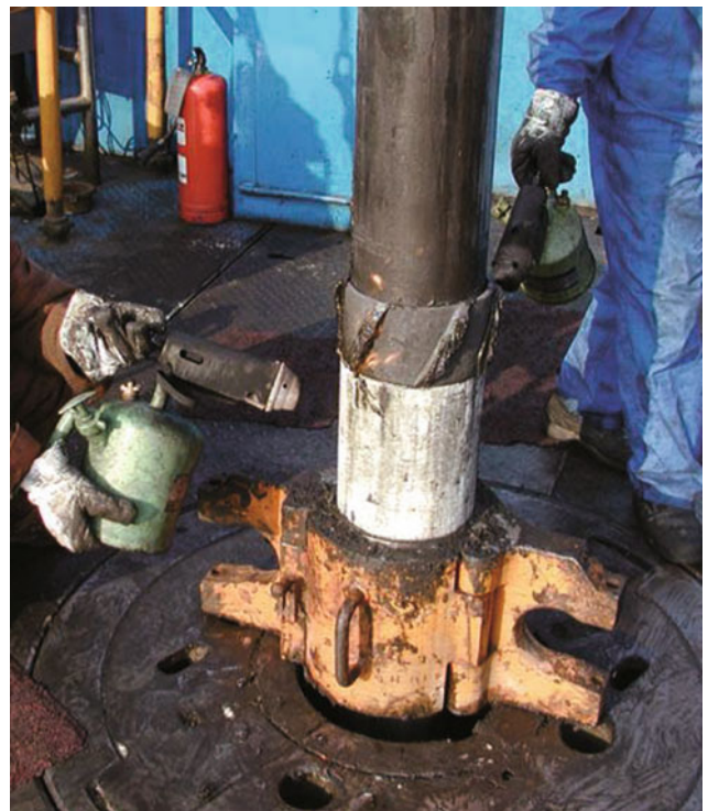
Fig. 10.35 Pulling 193.7 mm moving casing
