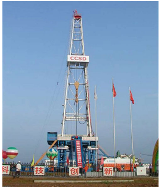
Fig. 3.6 ZJ70D drill rig used for CCSD-1 Well
