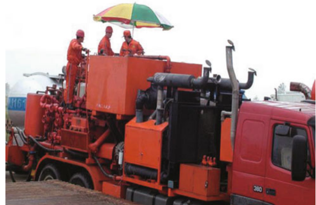
Fig. 10.19 Operation of 193.7 mm casing cementation
