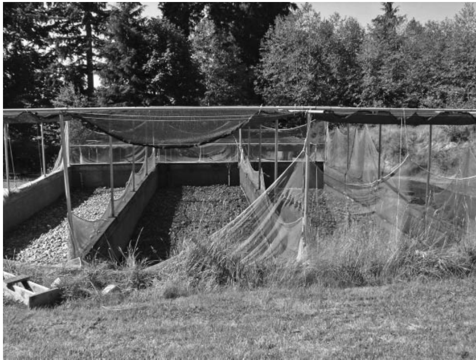
Figure 8.1. Spawning channels used for chinook salmon. These are approximately 4 m wide, 15 m long, and, when being utilized, are filled to a depth of between 0.5 m to 1 m, with continuous flow to mimic a stream environment. These channels have been drained to show the pebbles lining the bottom, which mimic the preferred spawning habitat of wild chinook in streams.
