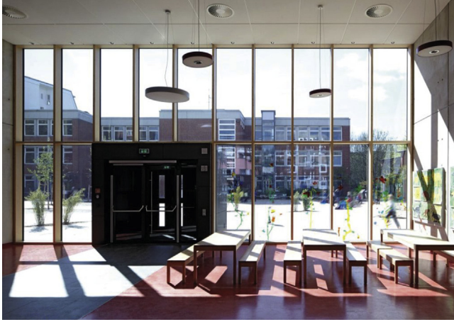
Figure 9.4 Electrochromic façade (clear). Courtesy of EControl-Glas GmbH.
