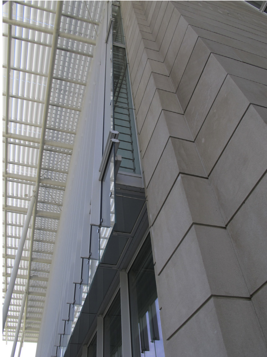
Figure 7.10 Glazed double-skin façade, exterior view, Chicago Art Institute, RPBW, Chicago. Photo by the author.
