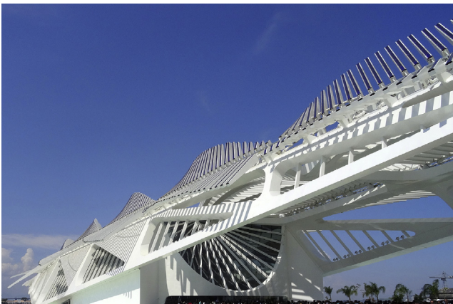
Figure 8.23 Museu do Amanhã, detail of PV-integrated movable roof components. Courtesy of Santiago Calatrava llc ©.
