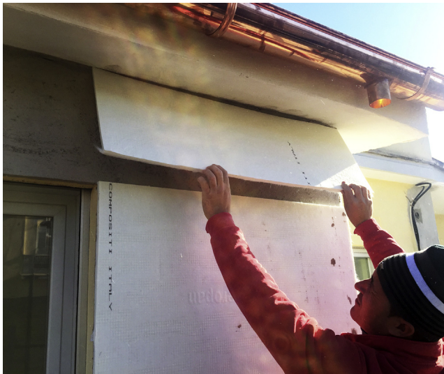
Figure 4.17 Aeropan installation.
