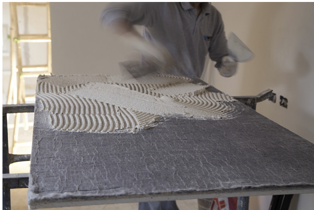
Figure 4.19 Installation of Aerogips panels. Courtesy of AMA Composites s.r.l.
