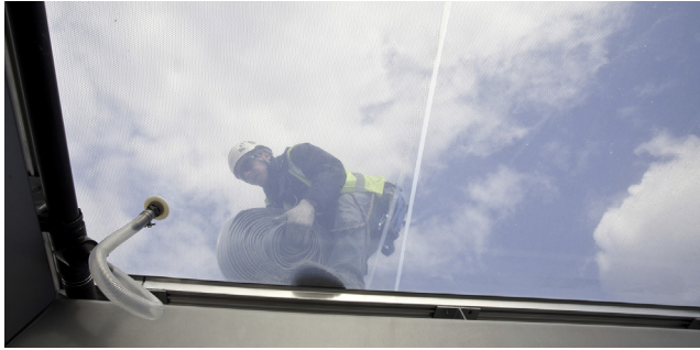
Figure 7.27 Detail of ETFE roof pressured air distribution, King's Cross Station, London. Courtesy of John Sturrock/Vector Foiltec ©.
