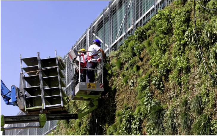
Figure 6.8 Green wall module installation. Courtesy of Peverelli s.r.l.
