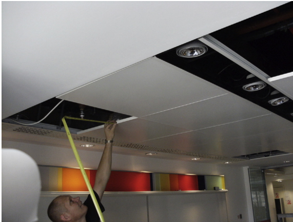
Figure 5.18 ThermoCool ceiling tile installation. Courtesy of Datum Phase Change Ltd.
