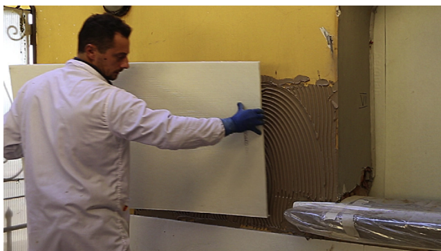
Figure 4.20 Installation of Aerogips panels. Courtesy of AMA Composites s.r.l.
