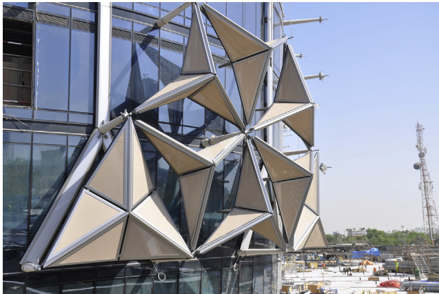
Figure 8.20 Al Bahar Towers dynamic shading system. Courtesy of Arup.
