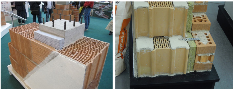
Figure 3.3 Thermal bridge correction and insulated cavity wall.
