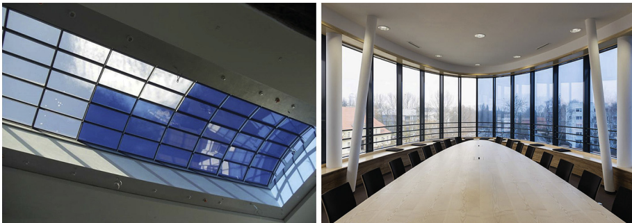
Figure 9.8 Electrochromic dynamic glazing. Courtesy of EControl-Glas GmbH.
