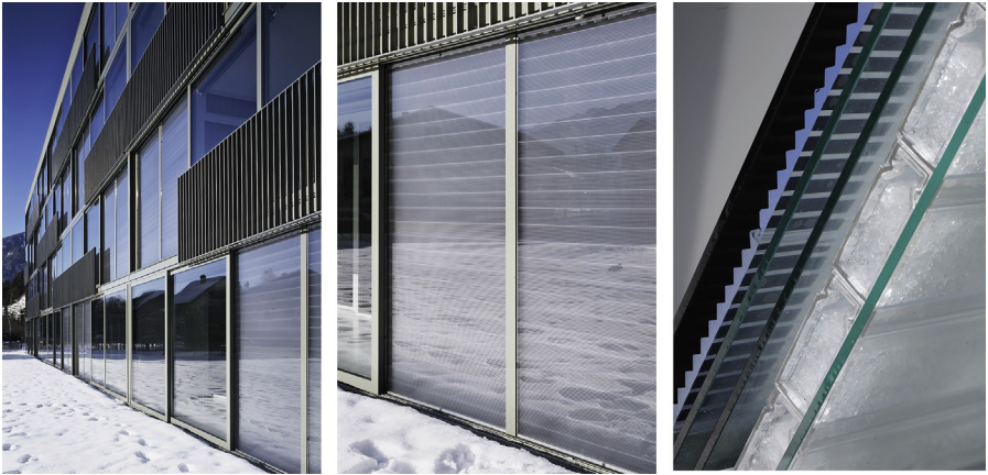
Figure 5.26 Retirement residence community, Schwarz Architekten, Domat Ems CH (left and center), and GlassX phase-change material glazing section (right). Courtesy of Gaston Wicky Photography ® and GlassX AG.
