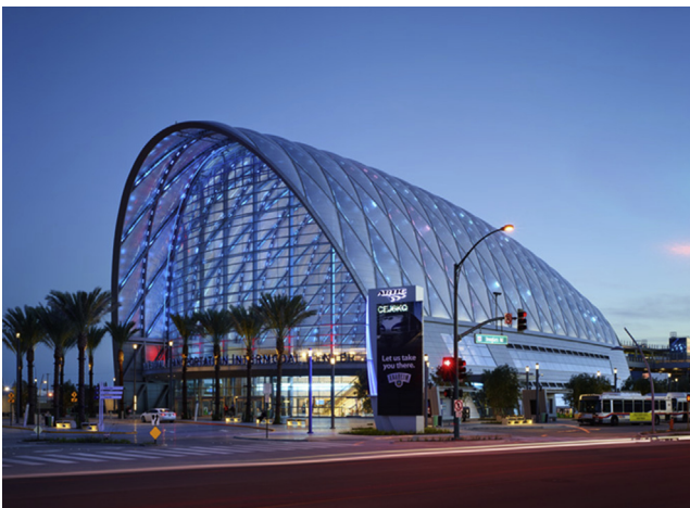
Figure 7.22 Anaheim Regional Transportation Intermodal Center, HOK, Anaheim, CA. Courtesy of John Linden/Vector Foiltec ©.
