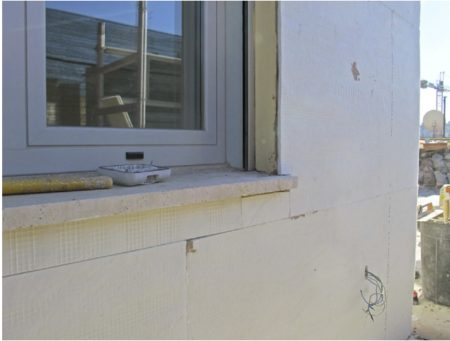
Figure 4.18 Installed Aeropan. Photo by the author.
