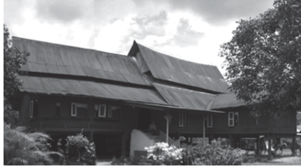
Fig. 18.3 Curved roof of Negeri Sembilan traditional house is adopted from the shape of a boat
