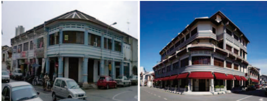
Fig. 45.2 Hutton road before and after rehabilitation works
