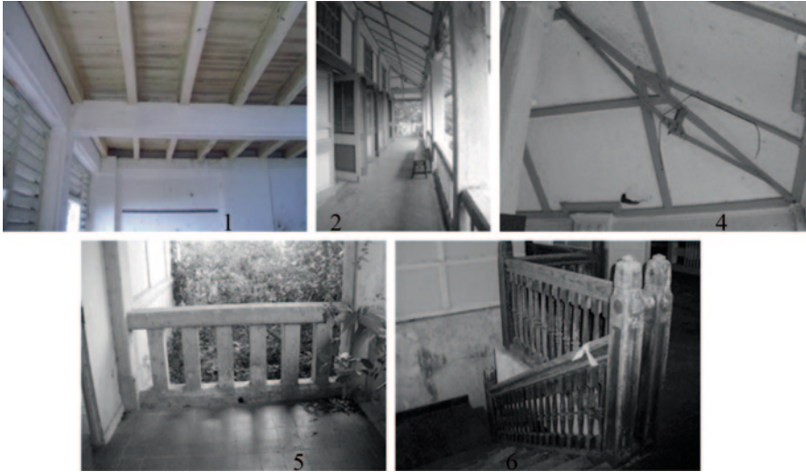
Fig. 43.3 The architectural elements of Crag Hotel: 1 timber floor boards and hardwood timber floor joists, 2 wide verandah, 3 vertical narrow window panes, 4 steel structure, 5 stone baluster, 6 hardwood timber staircase
