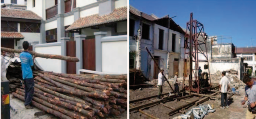
Fig. 45.7 Bakau piles and piling frame
