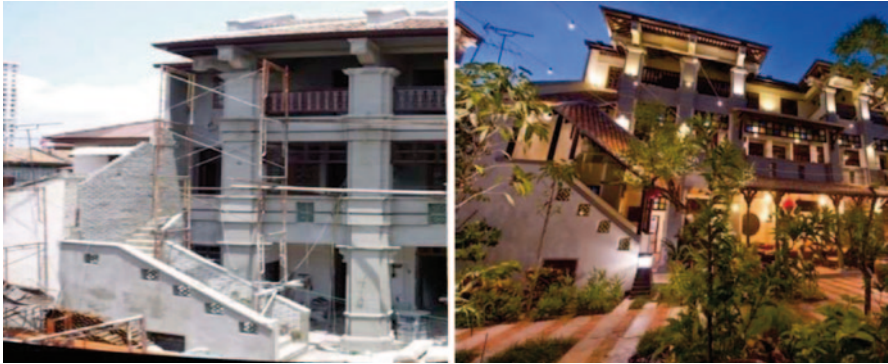
Fig. 45.9 Staircase under construction and staircase completed
