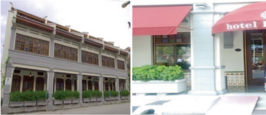
Fig. 45.13 Planter boxes at 5-ft way of Clarke terrace house
