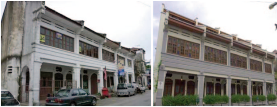
Fig. 45.4 Clarke road before and after rehabilitation works
