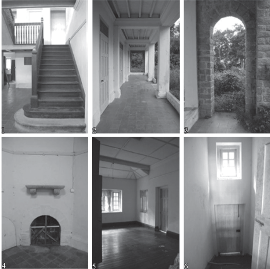
Fig. 43.4 The architectural elements of Woodside Cottage: 1 the hardwood timber staircase, 2 the wide verandah, 3 the masonry archway, 4 the fireplace, 5 high floor to ceiling heights, 6 volumetric space and a door with high level opening
