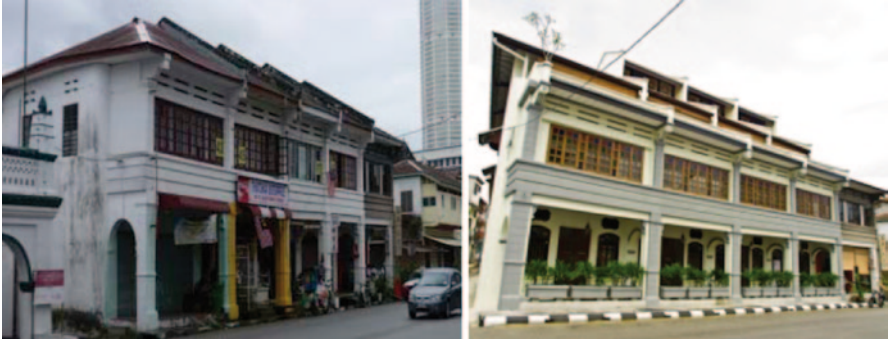
Fig. 45.3 Transfer road before and after rehabilitation works
