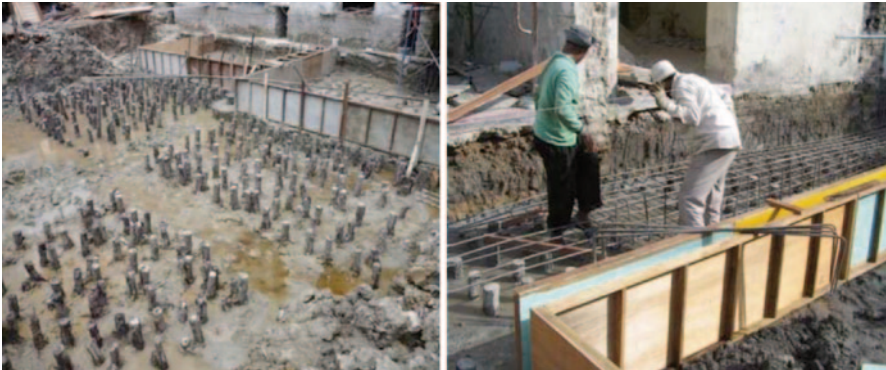
Fig. 45.8 Bakau piles piled and cut and steel rebar and footing formwork
