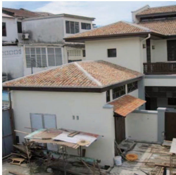
Fig. 45.14 TNB room under construction
