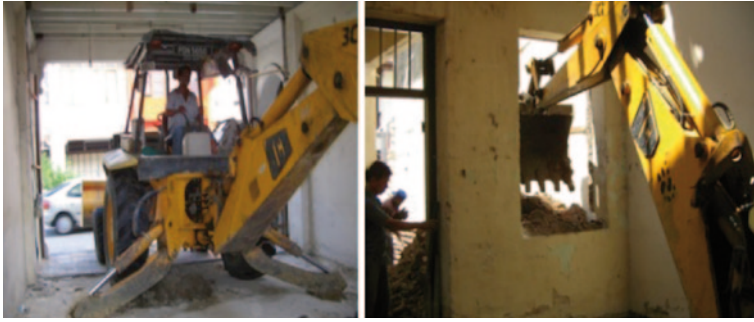
Fig. 45.15 Examples of tight working space
