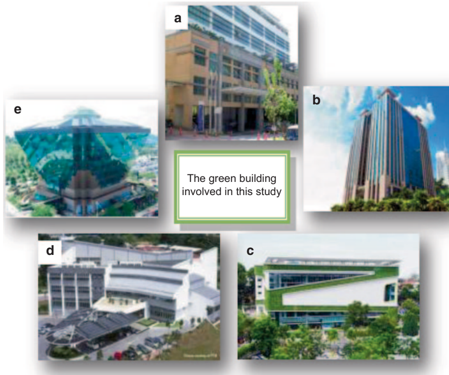
Fig. 31.1 a LEO Building, Putrajaya. b GTower. c DIGI Technology Operation Centre, Shah Alam. d GreenTech Malaysia, Bangi. e Diamond Building, Putrajaya
