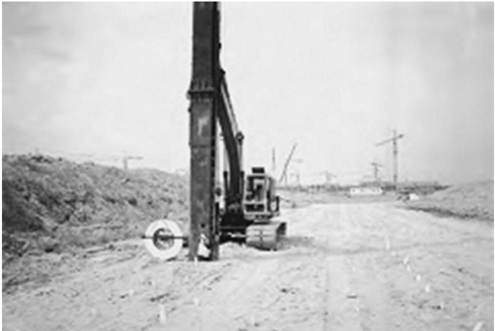
Figure 3.19 Installation of PVDs in the field (from Das, 2011).
