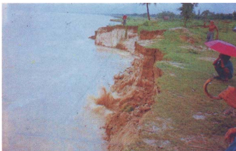
Plate 1 Bank erosion near Panchnandapur in Malda district (See also Photograph 5.1 on page 49)
