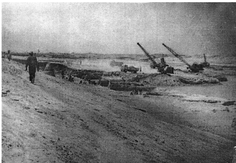
Photograph 7.7 Excavation of Feeder Canal in progress (1966)
