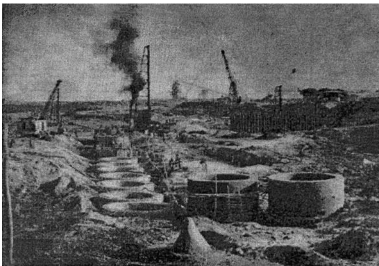
Photograph 7.5 Well sinking on right bank of Farakka, March 1965
