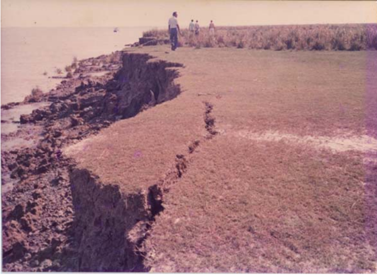
Plate 5 Bank slip of Nayachara island near Haldia (See also Photograph 5.5 on page 58)
