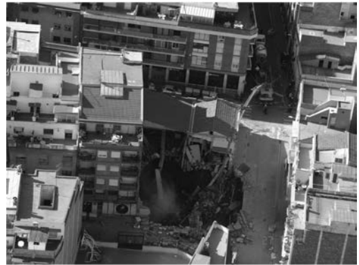
(b) Surface collapse
