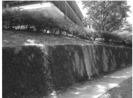
Figure 5. Photograph of blocked weep holes on a retaining wall taken by a student.
