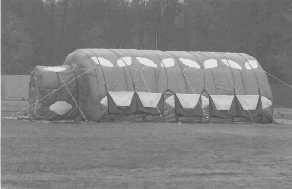
Figure 8.7. An inflatable habitat that may be used to construct a Mars base. Image courtesy: NOAA.
