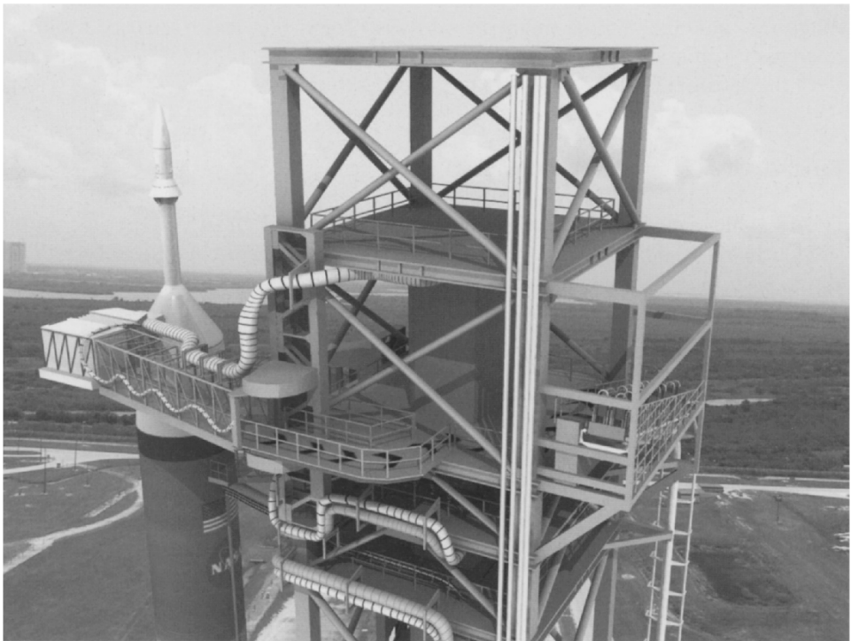
Figure 10.2. NASA's new emergency escape system. Note the rollercoaster system in the right of the image. Image courtesy: NASA.
