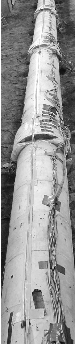
14.2 Reinforced concrete gravity pipeline with bell-and-spigot joint.
