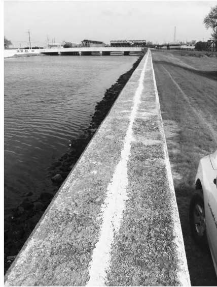
13.6 Installation of distributed FO strain-sensing cables on top of a retaining wall section in New Orleans Louisiana to detect wall movements. ( Source: Images courtesy iLevee Project, SMARTeC, Geocomp, Shannon & Wilson, New Orleans Levee District.)
