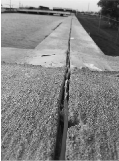
13.6 Installation of distributed FO strain-sensing cables on top of a retaining wall section in New Orleans Louisiana to detect wall movements. ( Source: Images courtesy iLevee Project, SMARTeC, Geocomp, Shannon & Wilson, New Orleans Levee District.)
