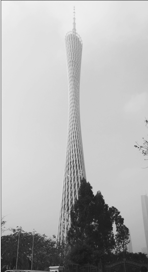
9.1 The Canton Tower (CT).
