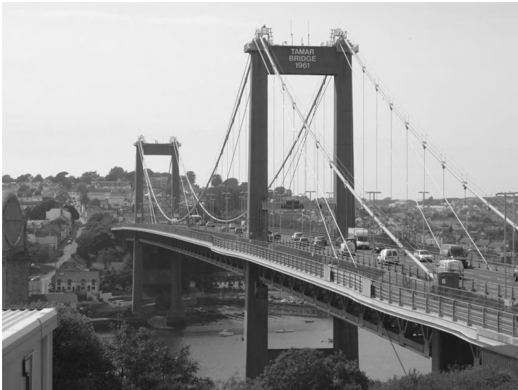
7.1 Tamar Bridge before and after strengthening and widening.
