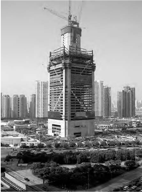
Figure 13.13 Construction of the World Financial Centre, Shanghai, China.
