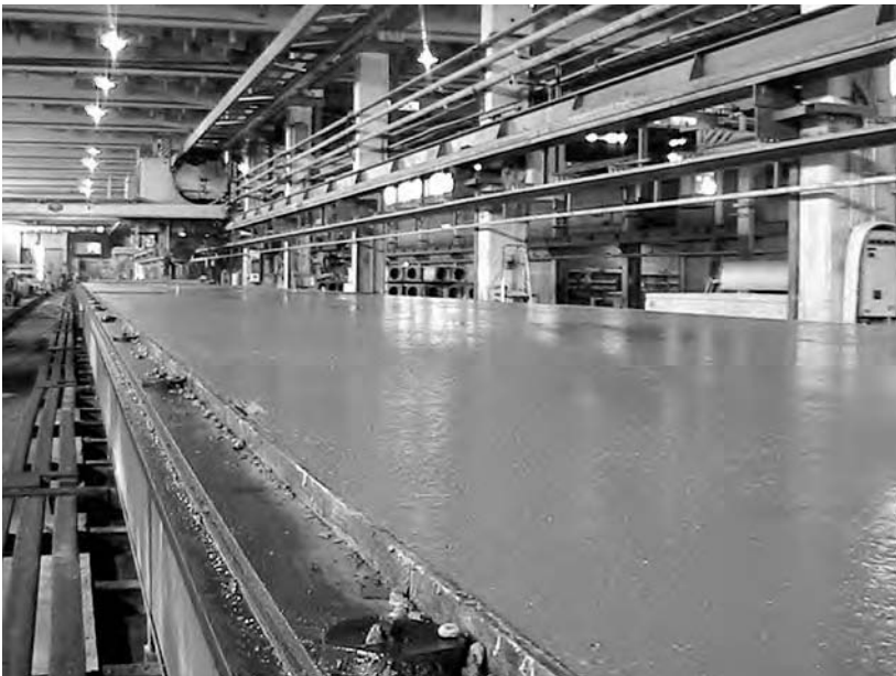
Figure 13.7 Surface of a prestressed slab after casting and finishing [3] .
