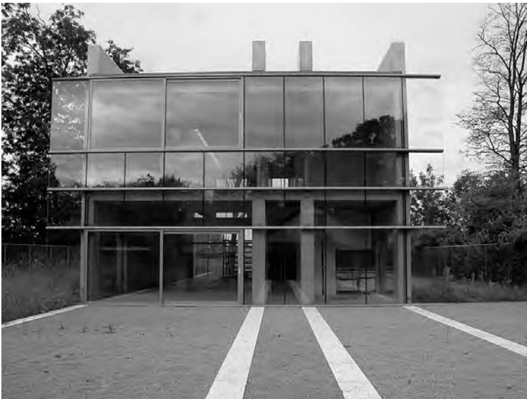
Figure 13.15 Villa in Gistel, Belgium. (Reproduced with permission of Engineering Office Mouton, Ghent, Belgium.)
