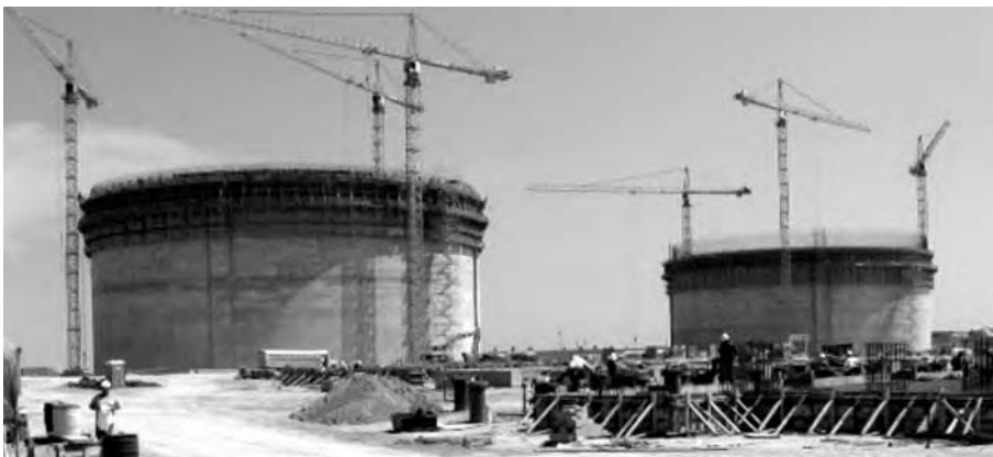
Figure 13.2 The two SCC Freeport LNG tank walls under construction [1] .
