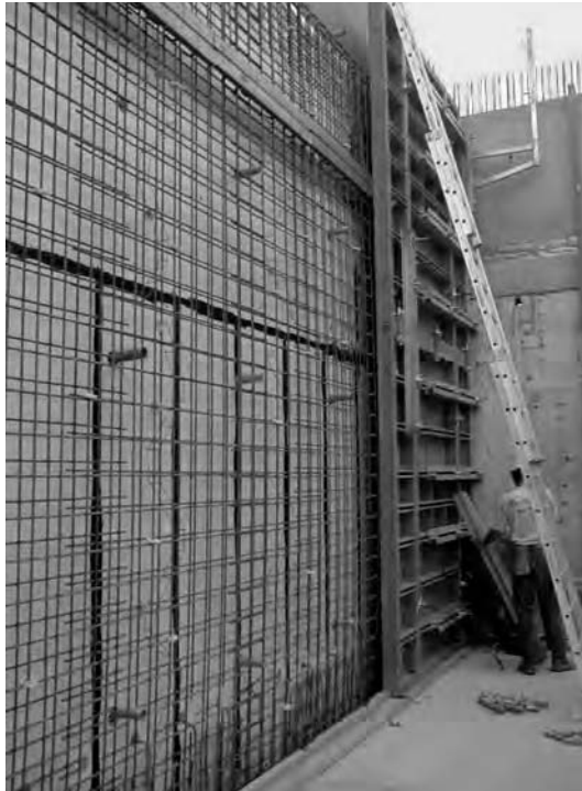
Figure 13.3 8 m high formwork for an industrial hall.
