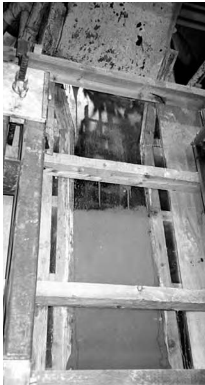
Figure 9.2 Full-scale structural elements (3 m tall columns) cast from SCC and TVC using crane and skip.
