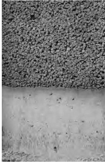
Figure 2.6 A single batch of a traditional low-medium slump concrete was used to cast the whole of this wall element. The bottom part was compacted by poker vibrators, the top part was placed without any compaction.
