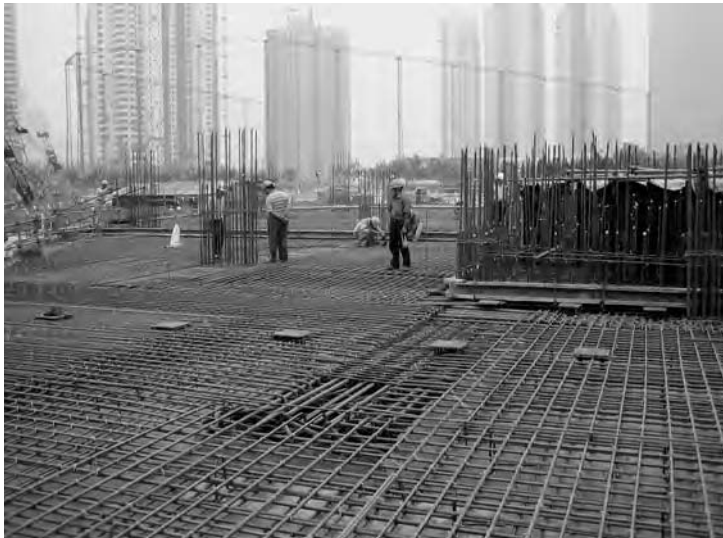
Figure 13.14 Foundation slab with dense reinforcement ready for casting.
