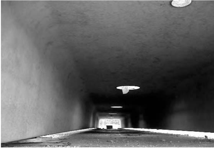
Figure 7.12 Excellent surface finish of large precast T-beams. (Reproduced with permission of C. Richards.)
