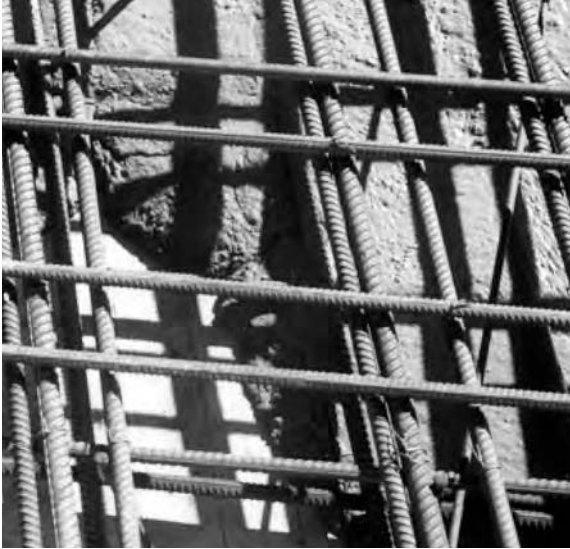
Figure 1.1 SCC flowing through a grid of reinforced bars.
