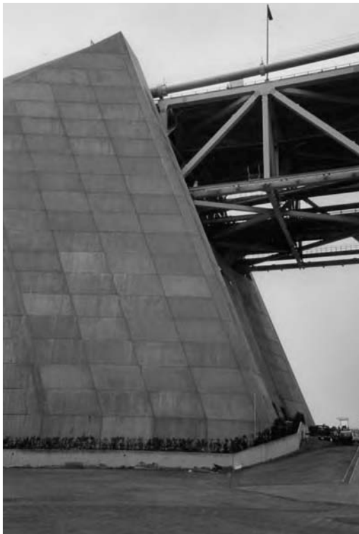
Figure 13.17 Southern abutment (height approximately 50 m) of the Akashi-Kaikyo Bridge, Japan.
