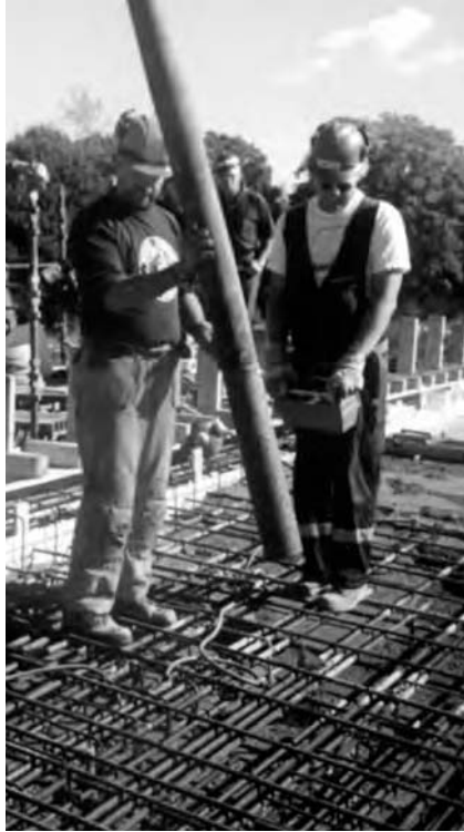
Figure 13.18 Casing of one of Europe's first SCC bridges, Nyneshamn, Sweden (1999).
