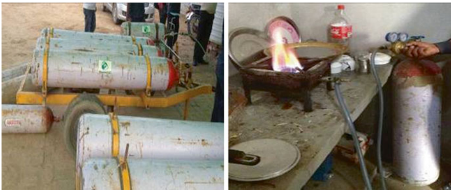
Fig. 13 Bottling of upgraded biogas in CNG cylinder cascade ( Left ) and bottled biogas being used for cooking ( Right )
