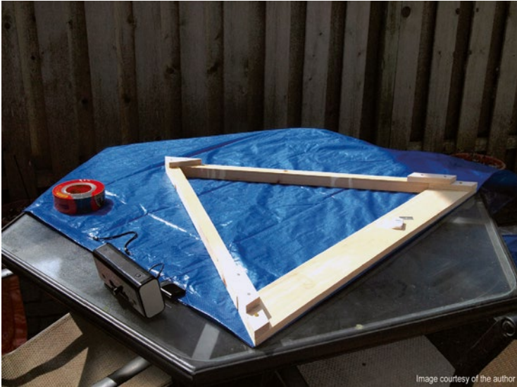
Fig. 5.23 Cutting the individual equilateral triangle panels from a sheet of tarpaulin material, which are ultimately taped together to form the skin of the dome
