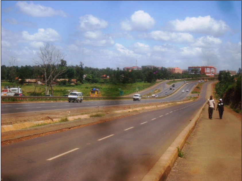
Photo 7.1: Thika Highway with service lanes and pedestrian walkway between Ruiru and Juja (Source: Author).
