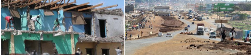
Demolitions of buildings along Thika Road (Source: Stephen Mudiari 2008, http://thm-a02.yimg.com/nimage/09cdd6df0f3715e6 ).
