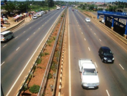
Thika Highway with matatu stop seen from footbridge (Thika to Juja)
