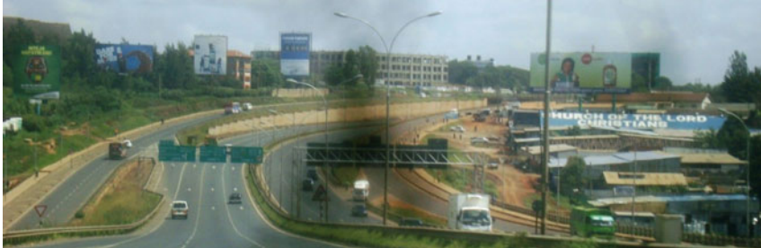
Thika Highway with service lanes and access roads through built-up area (Nairobi)
