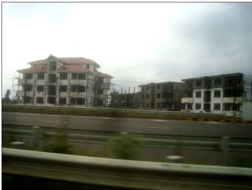
Photo 5.9: Construction of middle-income apartment blocks between Nairobi and Ruiru (Source: Author).
