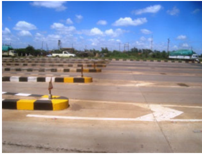
To-be installed toll station on Thika Highway (Juja to Ruiru)
