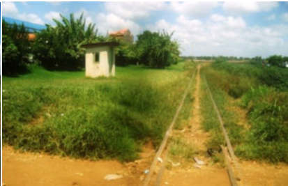
Rail track at the town periphery (Ruiru)
