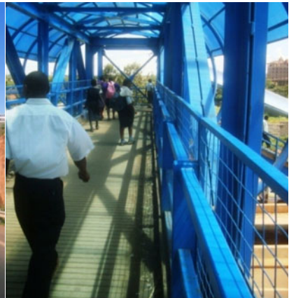
Afterwards installed footbridge (Ruiru)
