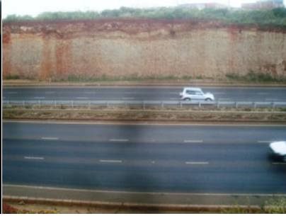
Thika Highway cutting through settlement (Witeithie)
