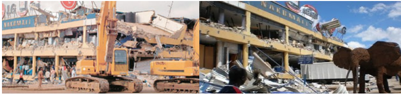
Demolition of the Thika Road Nakumatt store (Source: Joseph Mathenge 2008, http://www.nation.co.ke/image/view/-/486200/highRes/48914/-/maxw/600/-/ebmj8/-/Nakumatt.jpg ).
