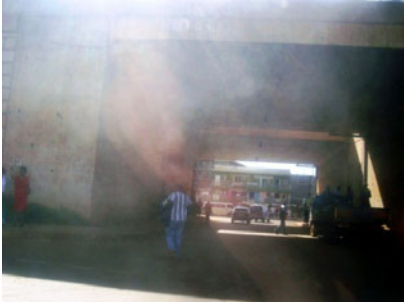
Pedestrians using underpass below Thika Highway (Juja to Thika)
