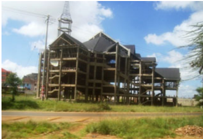
New church under construction (Thika)
