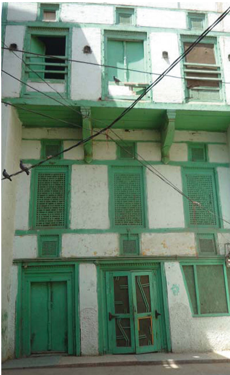
Fig. 18.2 Wooden frame and bricks
