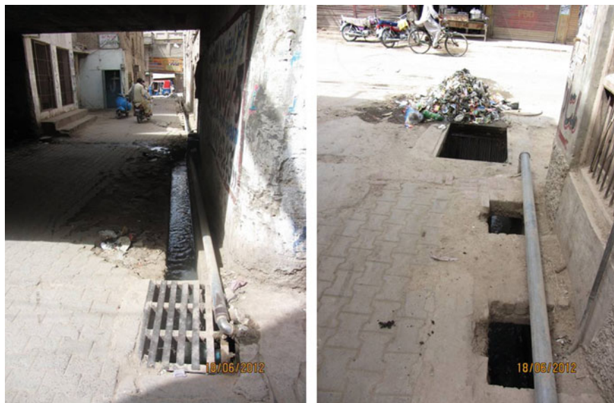
Fig. 12.2 Pictures of the project area. Left : the network underpasses the Alang Road bridge. Right : the connection with the circular road sewerage, with a large amount of solid waste
