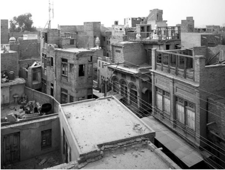
Fig. 1.2 View from the roofs in Multan (photo by M. Introini)
