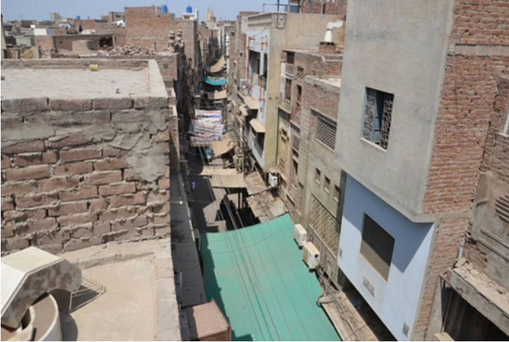
Fig. 10.3 An urban canyon in Multan. Buildings have irregular height and average H/W = 2
