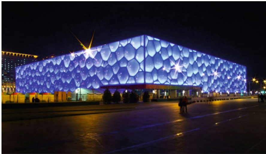
Fig. 4.7 Beijing National Aquatics Center (the Water Cube)
