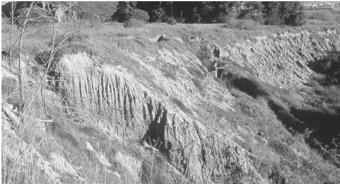
FIGURE 10-8. Site preparation is mandatory to ensure the wattles can effectively control erosion on the steep slope and prevent the formation of rills and gullies. Naval Base Point Loma, San Diego, California. (Photo by Mary F. Platter-Rieger.)
