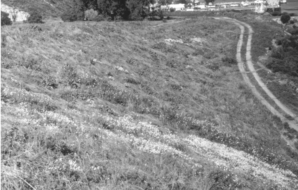
FIGURE 10-10. The same site in figure 10-9 after sixteen months: no significant erosion, wattles in good condition. Sprinkler irrigation was on an as-needed basis for the first twelve months. Naval Base Point Loma, San Diego, California. (Photo by Mary F. Platter-Rieger.)
