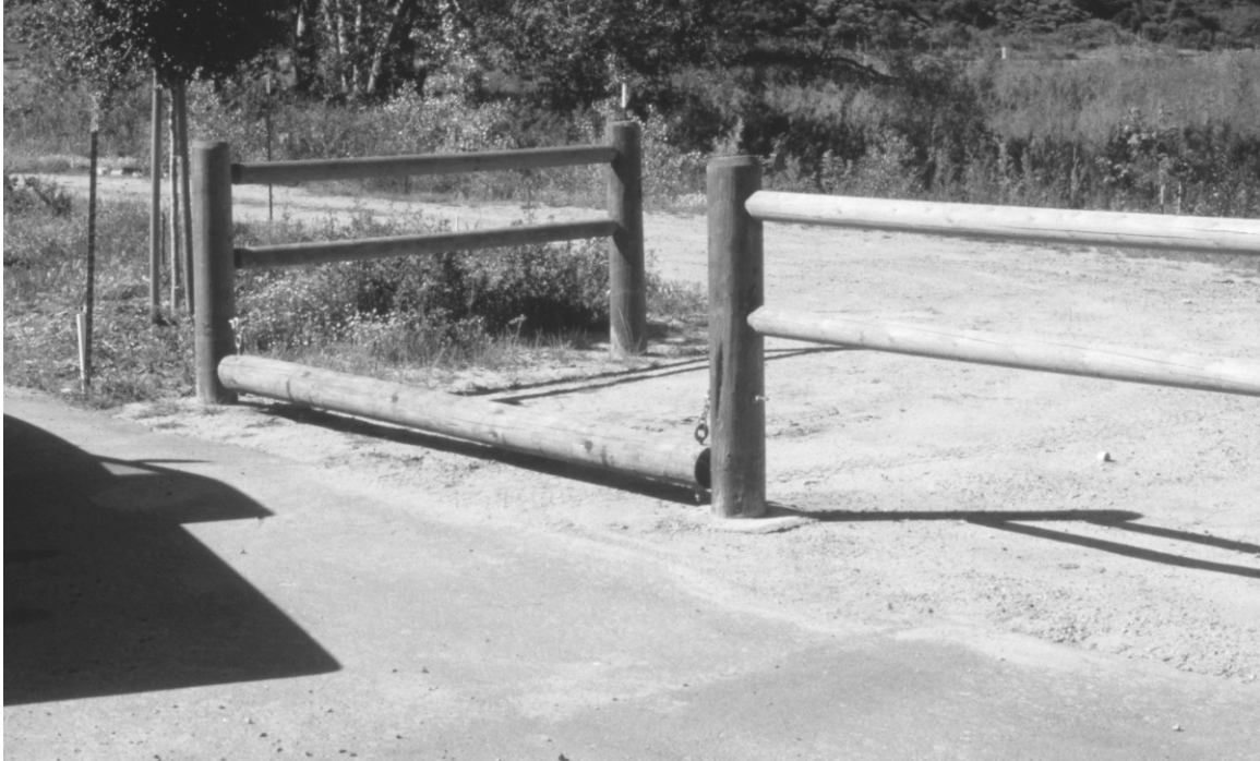
FIGURE 10-14. Access control for vehicle and motorcycle while allowing passage of bicycles, horse riders, and hikers. The hanging horizontal log moves away and up when pushed farther, thereby blocking passage. (Photo by John Rieger.)
