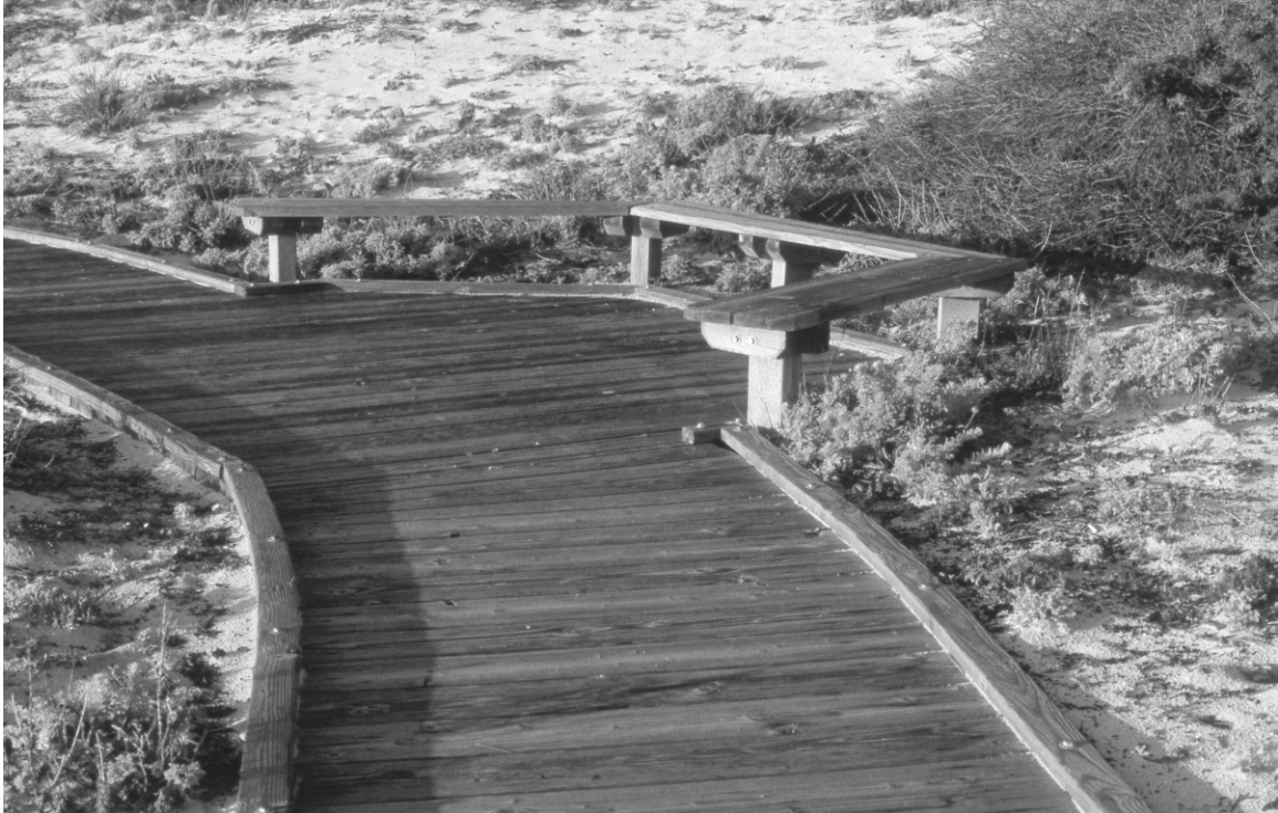
FIGURE 11-3. A boardwalk in this coastal dune complex has controlled wandering over the dunes, allowing vegetation to reestablish. Carmel, California. (Photo by John Rieger.)
