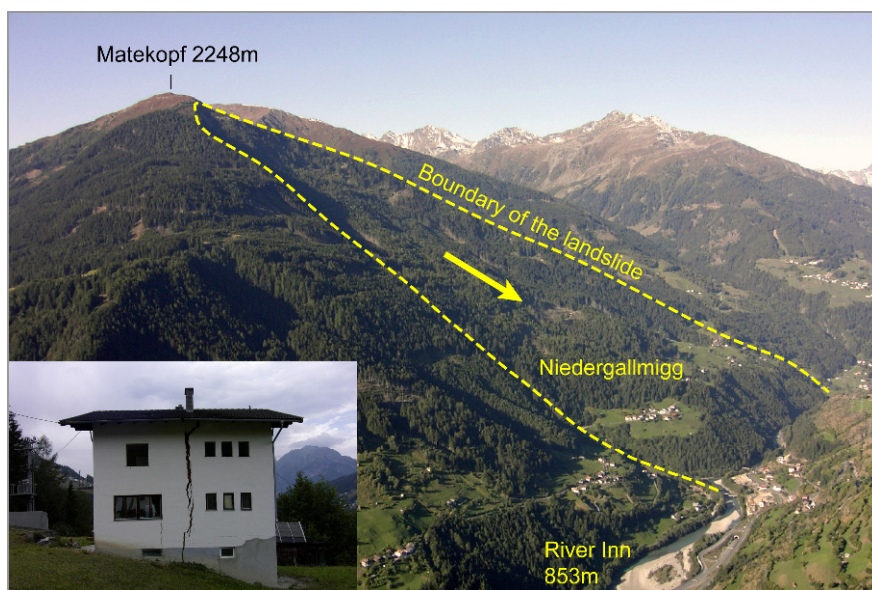
Fig. 5.15 View of the Niedergallmigg-Matekopf landslide. Insert shows movement induced fracturing of a house on the landslide
