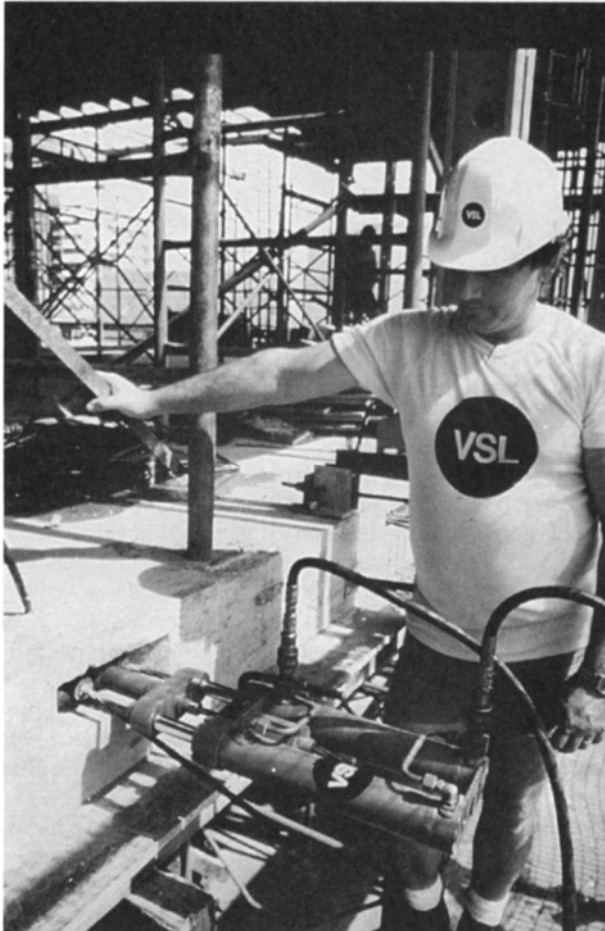
Figure 13.4 VSL mono jack (twin ram), stressing slab tendon, Australia
