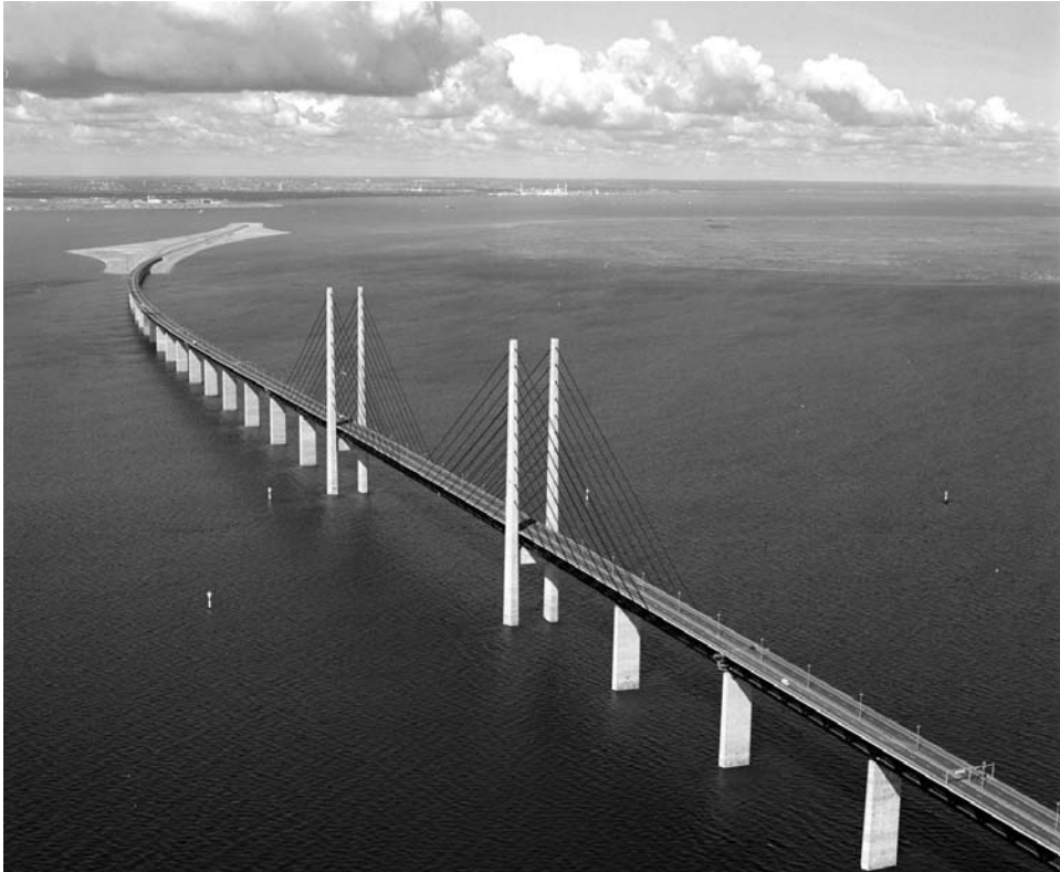
Figure 9.8. The Öresund bridge, seen from the east looking toward Copenhagen. (Courtesy of Bridgephoto, Denmark; http://bridgephoto.dk/search/start.php )
