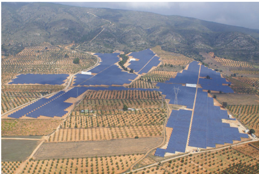
Fig. 1.6 A photograph of Beneixama 20 MW PV power plant [27]
