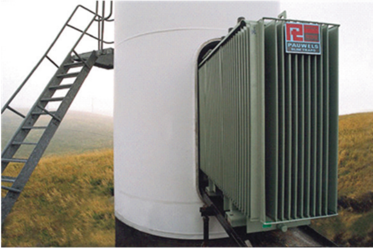
Fig. 7.18 A Pauwels transformer being lifted through the door of a wind turbine tower during installation
