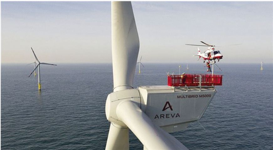
Fig. 1.5 A photograph of offshore wind farm under maintenance [25]
