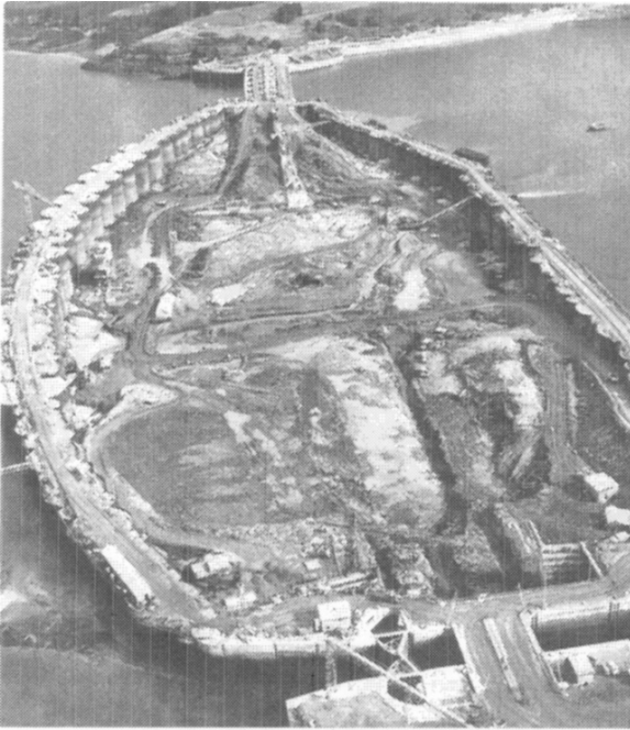
Fig. 4.3 Work proceeded at Rance River site inside cofferdams
