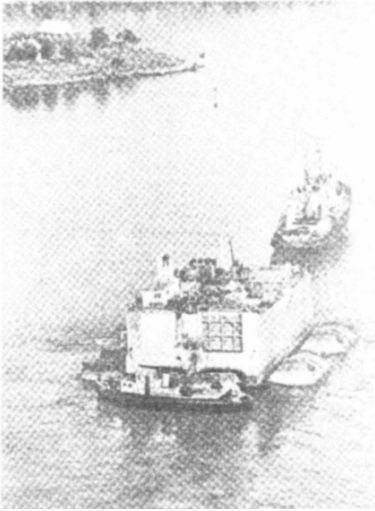
Fig. 4.12 Powerhouse being towed to site
