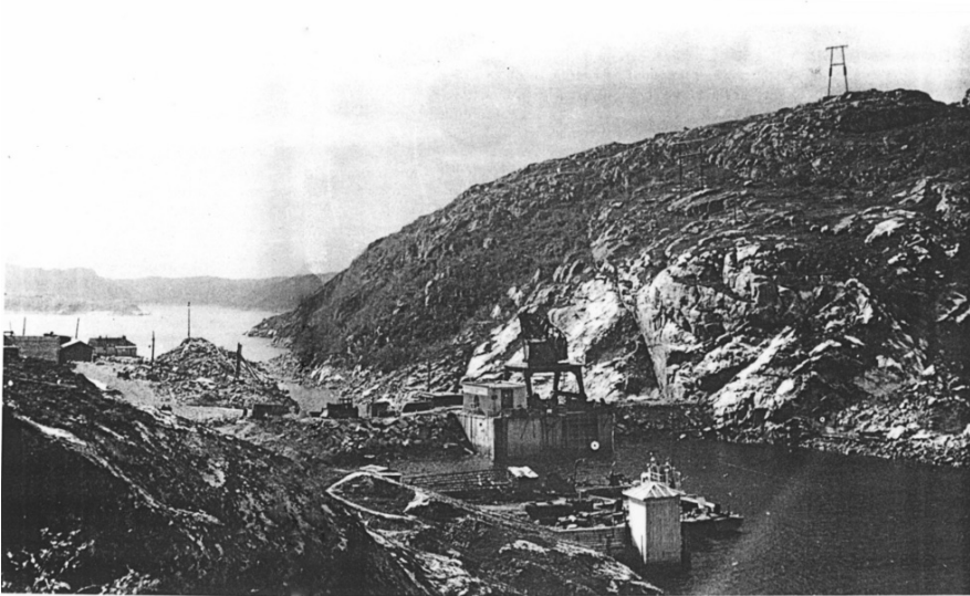
Fig. 4.9 View of the Kislaya Bay TPP
