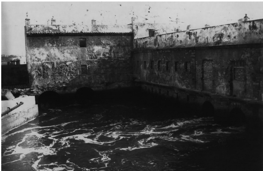
Fig. 2.10 (b) Arillo tide mill located on road to Cadiz, new facing the sea. (figs. 2.10 belong to Archives of French Land-forces, now in Vincennes, France) (c) Present condition Arillo tide mill. (Photo L. Ménanteau)
