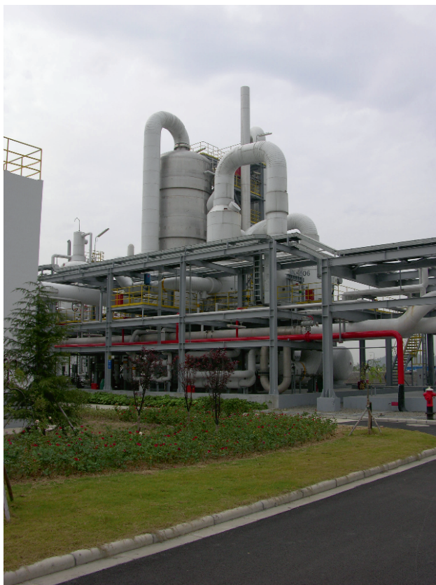
Figure 4.9. Plant for the manufacture of formaldehyde by metal-oxide-catalysed process. Photograph by Stan Erismann, Per-stop Formex.
