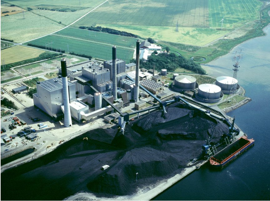
Figure 11.1. Coal-fired power plant fitted with SCR (Selective Catalytic Reduction) unit to decrease NO x content of the flue gas. Reproduced with permission from Haldor Topsøe A/S.
