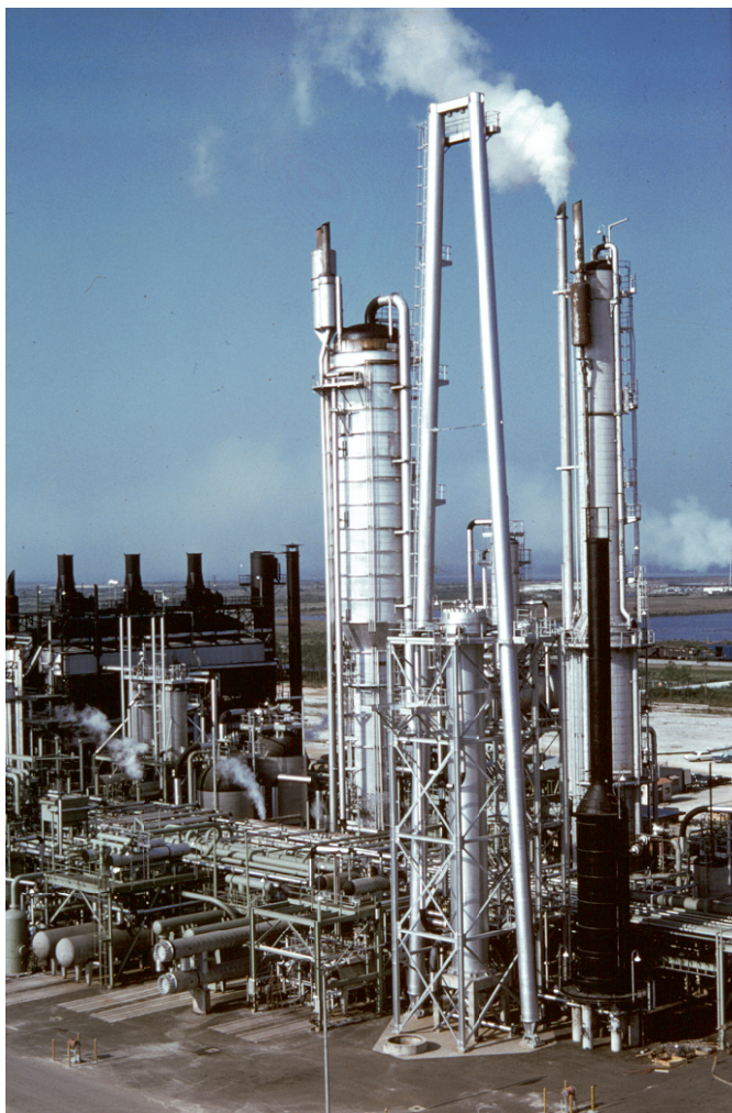
Figure 10.7. Topsøe converters for ammonia synthesis. Reproduced with permission from Haldor Topsøe A/S.
