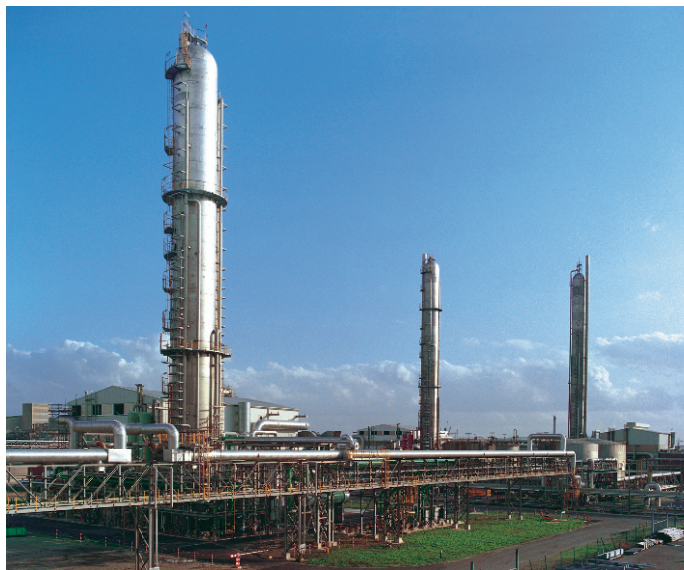
Figure 4.1. A typical modern plant for the manufacture of nitric acid. Reprinted with permission from Uhde GmbH.
