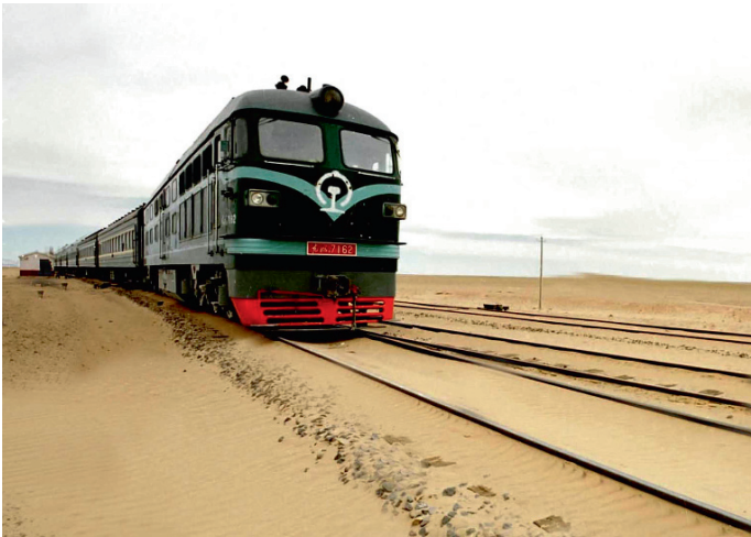
Fig. 1.5. A photo of the Jining-Erlianhot railway threatened by the invaded shifting sand. On May 29, 2002, an international train from Beijing to Ulan Bator, Mongolia, driving on the railway threatened; the Jining-Erlianhot railway is an important component of Eurasian Continental Bridge, but the shifting sand threatens the transportation safety (Xinhua News Agency)
