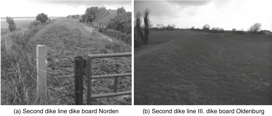
Fig. 2.9 Second dike lines in Lower Saxony
