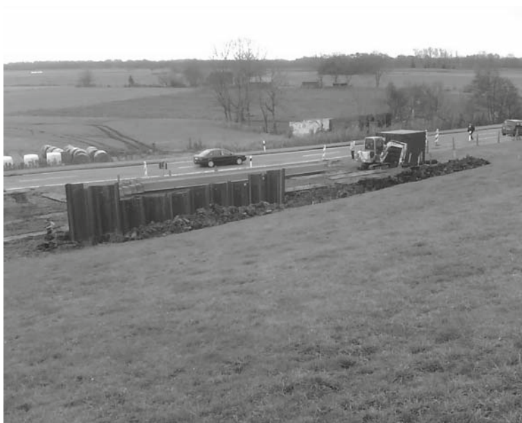
(b) Sheet piles on the inner slope
