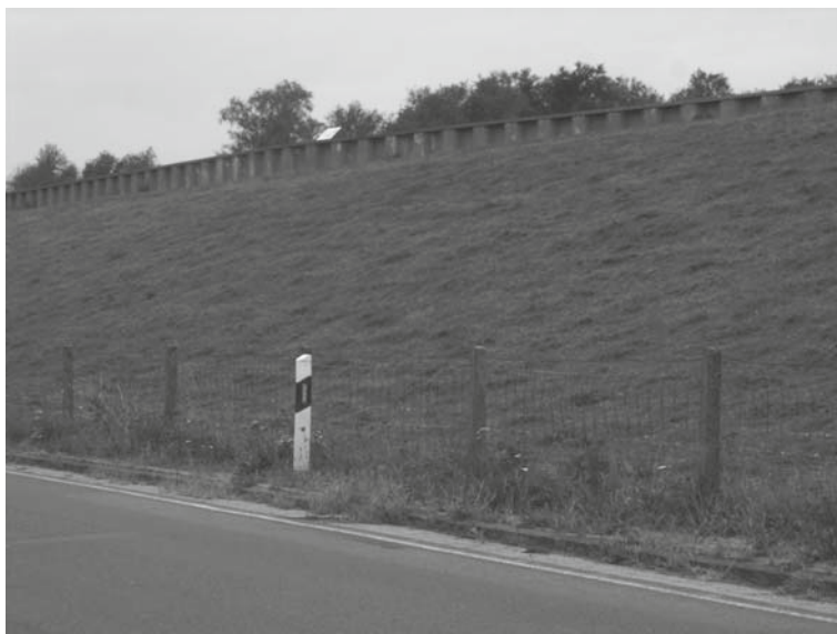
(a) Sheet piles on the dike crest
