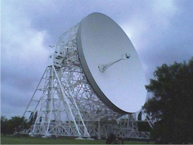
Fig. 1.3 The Lovell radio telescope (formally the Mark 1) at Jodrell Bank Cheshire in the United Kingdom (This image was taken shortly after the surface of the dish had been recently replaced with a more accurately shaped and smoother surface which allowed the telescope to be used at even higher frequencies. Also at the time the image was taken the structure was having a fresh coat of paint)
