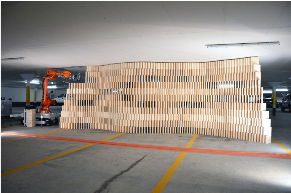
Fig. 3. An 8-metre-long modular wall, digitally fabricated in the parking garage of the Department of Architecture at ETH Zurich using an additive assembly method, for which the robot had to reposition itself several times (Gramazio & Kohler, ETH Zurich, 2012)
