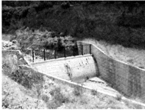
Figure 8. Existing sediment control structure upstream of the highway crossing.
