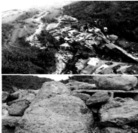
Figure 4. During typhoon Troaji period, a large amount of boulders deposited in the village upstream and
