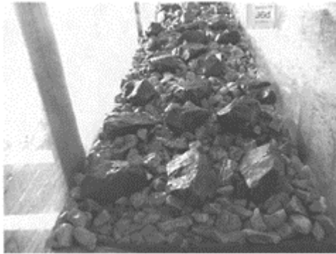
Figure 5. Boulders placed over the ramp (upstream view).
