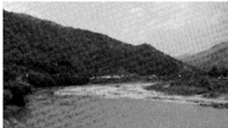
Photo 7. Floodplain in Kawasaka district after the flood.
