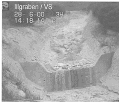
Figure 2. Debris flow front for the 28 June 2000 event from the video tape. The base width of the check dam is about 10m. Mud traces from an earlier event in summer 2000 are still visible immediately downstream of the front.
